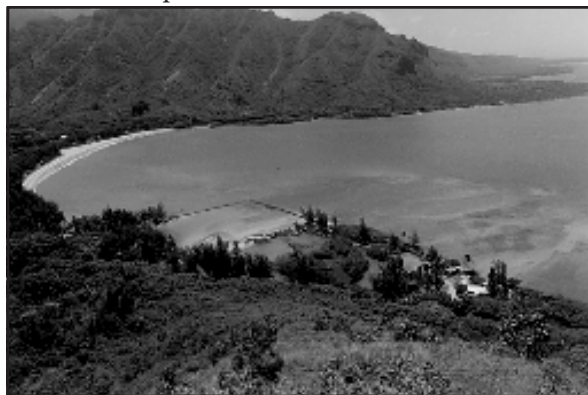
Huilua Fishpond in 1980 with wall damage.
