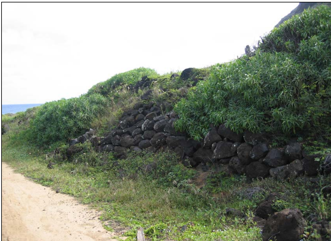
Fig. 26: Rock Retaining Wall along Mauka Edge of Railway Bed near Northern Bend in the Alignment (Facing Northwest). Note use of water-worn stones.
