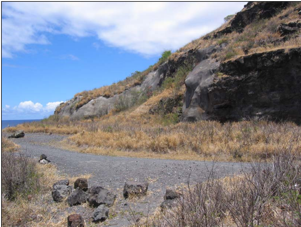
Fig. 32: Sealed Entrance to BCN-409 Northern Tunnel (Facing Northeast). Note Ridge Cuts Stabilized with Pressure-Sprayed Gunite.
