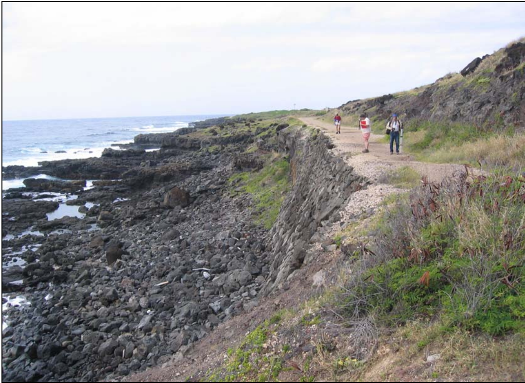
Fig. 21: Rock-Faced Retaining Wall for Railway Bed Southeast of the Project Area (Facing Northwest)
