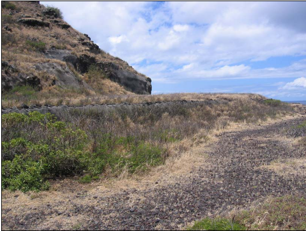
Fig. 33: Edge of Terraced, Cut and Fill Road Bed Stabilized with Pressure-Spray Gunite (Facing Southeast).
