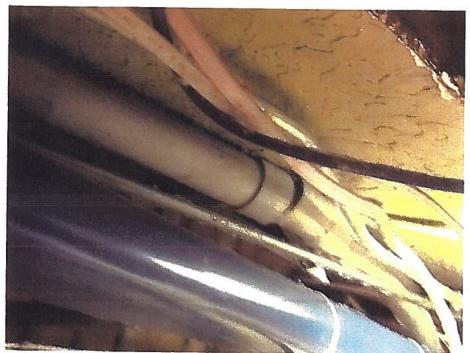
Storage room ground floor next to electrical room in between West and South wing. Feeder PVC conduit coupling has come apart exposing energized conductors. (358.42 Couplings and Connectors). Couplings and connectors Used with EMT shall be made up tight.
