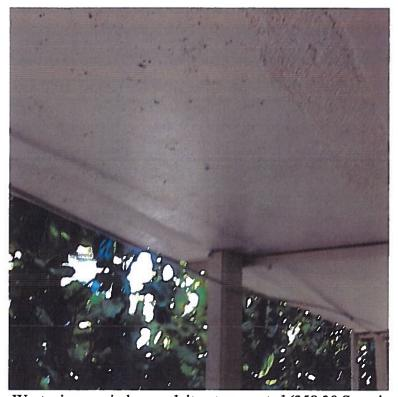
West wing corrigdor conduit not supported (358.30 Securing and Supporting)
