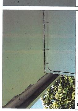
Photo 64. Depicts close up of deteriorating concrete roof overhang and cracking of the wall/roof of the West wing.
