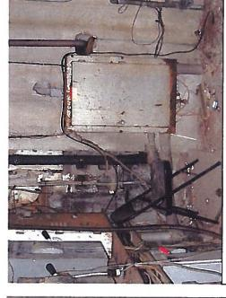
Photo 24. Depicts interior of electrical room. (no fire separation, pipe penetrations not protected)
