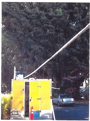
(230.26 Point of Attachment). In no case shall this point of attachment be less than 3.0 m (10 feet) above finished grade.
