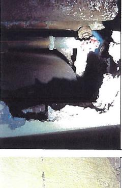
Photo 48. Depicts leak at tub drain in a room on the ground floor in the North wing.
