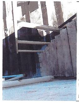
Photo 42. Depicts non-code compliant stairway on the roof of the East and North wing.
