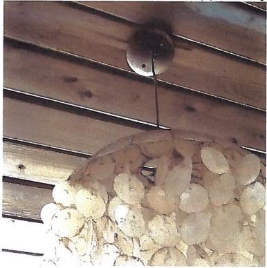
Fixture in resturaunt dining area supported only by flexible cord (400.10 Pull at Joints and Terminals) Flexible cords and cables shall be connected to devices and to fittings so that tension is not transmitted to joints or terminals.
