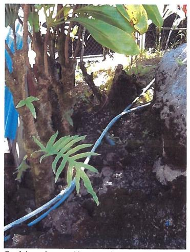
Conduit used exposed in areas of physical damage shall be identified for the use. Type Schedule 80, is identified for areas of physical damage.
