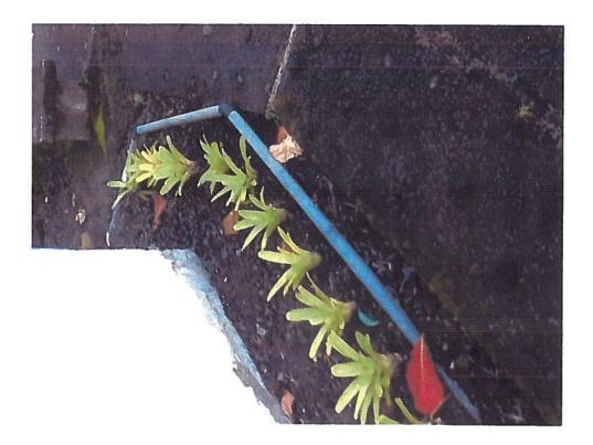
Conduit used exposed in areas of physical damage shall be identified for the use. Type Schedule 80, is identified for areas of physical damage.
