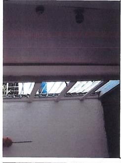
Photo 73. Depicts non-code compliant guardrail at window in the corridor of the North wing.
