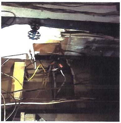
(In Lobby Electrical Room) Junction box with no cover now exposes energized conductors) (334.15 Exposed Work
