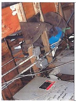
Photo 25. Depicts ceiling of electrical room. (Faulty weather protection, leaking roof)
