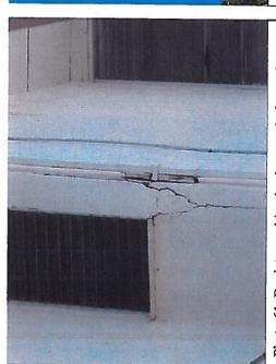
Photo 61. Depicts cracking in elevator shaft exterior wall.
