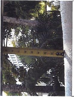
Photo 36. Depicts spacing in guardrail at units in the East wing.
