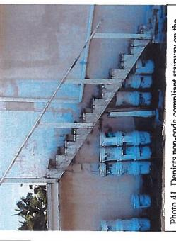
Photo 41. Depicts non-code compliant stairway on the roof of the East and North wing.
