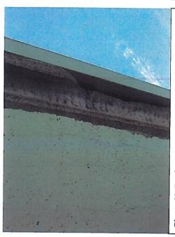
Photo 65. Depicts close up of deteriorating concrete roof overhang of the West wing.
