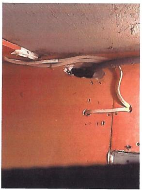
West wing corridor storage room use of NMB cable without protection (334.15 Exposed Work. (B) Protection required from Physical Damage)
