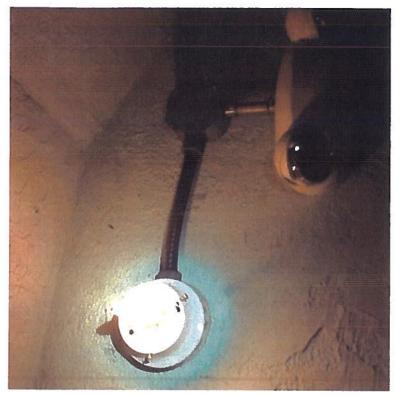
(East Wing typical Stairway lighting 1-4 floors) light fixtures with no covers to protect lamps from accidental contact.
