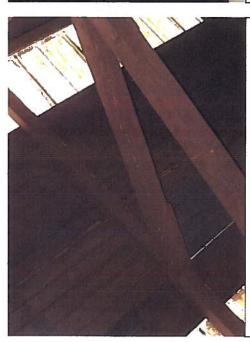
Photo 19. Depicts termite damage to roof deck and truss system in lobby area.
