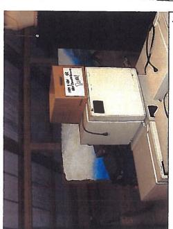
Photo 31. Depicts interior of unpermitted storage on  $2^{\rm nd}$  floor of East wing. (no fire separation between storage room and lobby)
