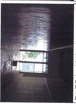
Photo 52. Depicts window in corridor open to exterior balcony of adjacent room. (no fire separation between corridor and room)
