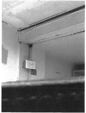
Laundry room ground level use of NMB cable. NMB cable without protection (334.15 Exposed Work (B) Protection from Physical Damage.)
