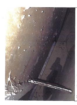
Photo 49. Depicts opening in floor ceiling assembly of ground and 1st floor in North wing. (no fire separation between floors)
