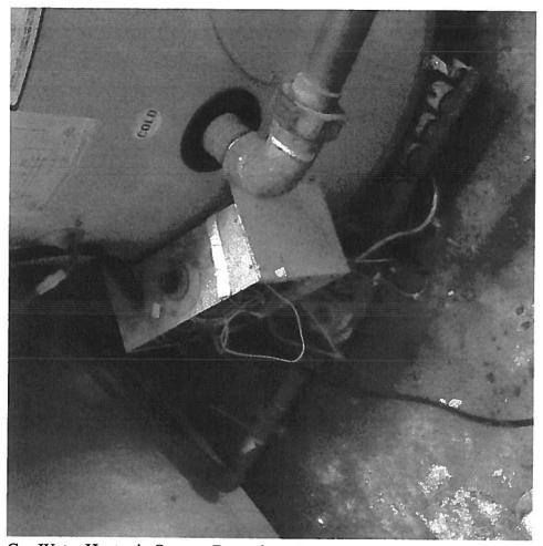
Gas Water Heater in Storage Room between North and East wing no cover on junction box energized conductors present.
