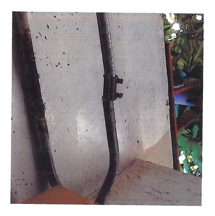
West wing corridor conduit not properly connected coupling not Connected. (358.42 Couplings and Connectors) Couplings and connectors used with EMT shall be made up tight. Where buried in masonry or concrete, they shall be concrete tight type. (Where installed in wet locations, they shall comply with 314.15.
