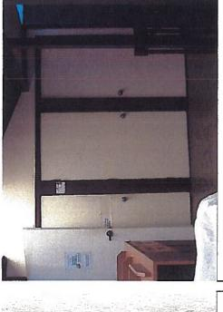
Photo 69. Depicts non rated doors to mechanical rooms in the lobby area. (no fire separation between mechanical room and lobby)
