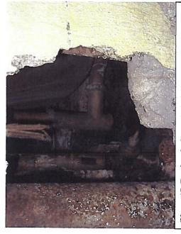
Photo 47. Depicts leak at tub drain in a room on the ground floor in the North wing.
