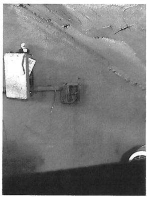
Pool room junction / device box uncovered and possibly Conductors may still be energized. (110.27 Guarding of Live Parts.)
