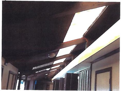
Fire alarm cable exposed in lobby area not listed to be run exposed 110.3(B)
