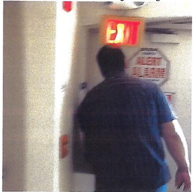
Exit light North wing corridor subject to physical damage Due to in proper mounting height 6'-6" (110.27 Guarding of Live Parts.)
