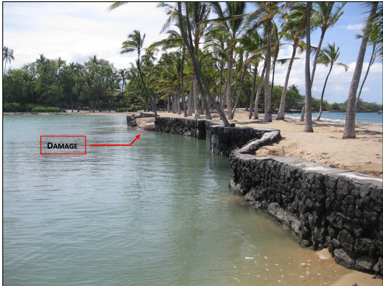
Figure 3-1 Existing Pond Wall
