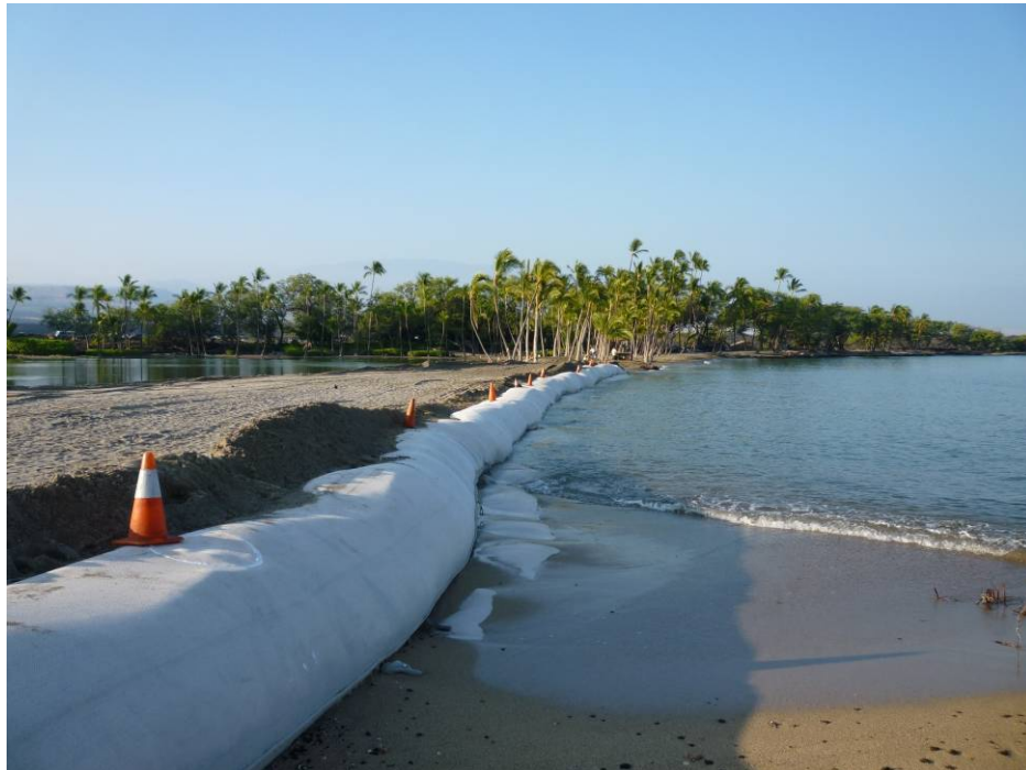
Figure 2-3 Post Emergency Repair, August 4, 2011
