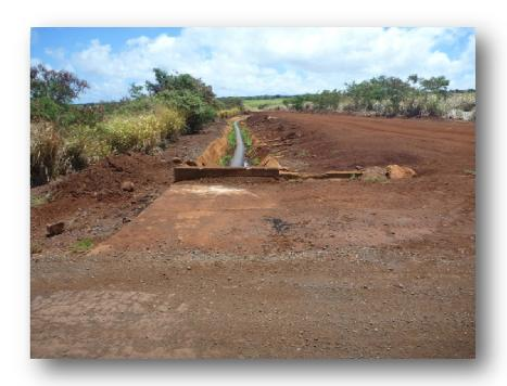
Plate 3. An irrigation ditch runs under 'Opae'ula Road through a concrete box culvert adjacent to the irrigation reservoir at Sampling Point O2.
