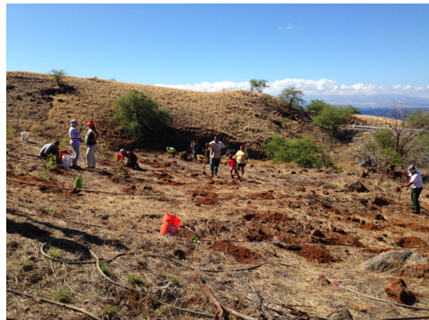
Figure 4.3: Volunteers helping install irrigation lines.
