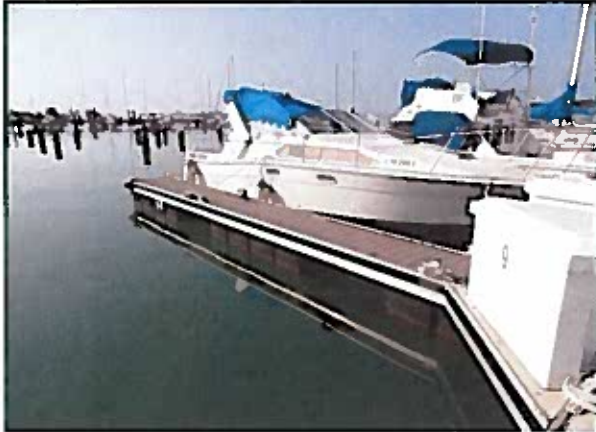
Representative view of a finger with a storage locker on a floating pier.
