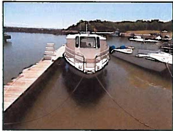
Representative view of a fixed catwalk of wood construction.
