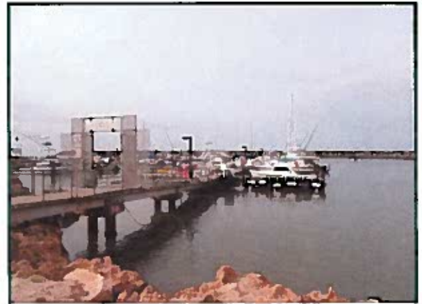
View of Pier C.
