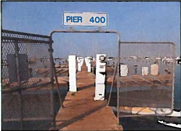
View of Pier 400, a fixed wooden dock.
