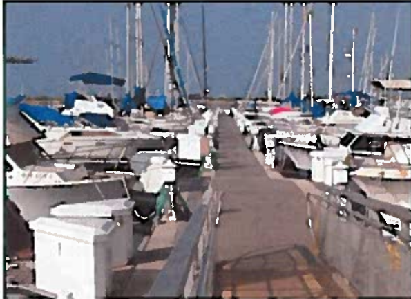
Representative view of a composite floating pier with storage lockers.
