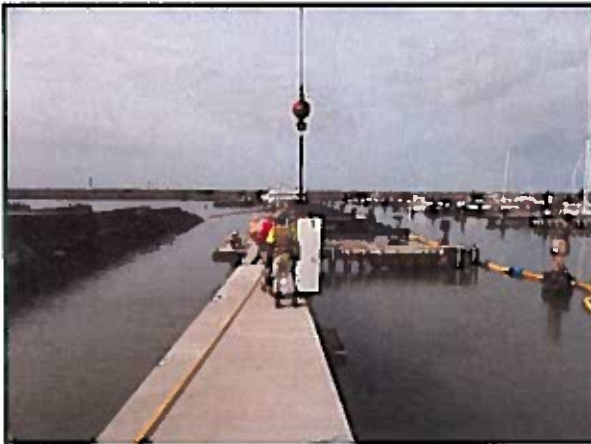
Pier A (under construction).
