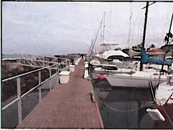
Newer composite fixed dock along breakwater with Tahiti moorings.
