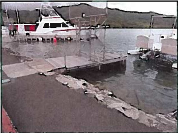
Representative view of a pier.
