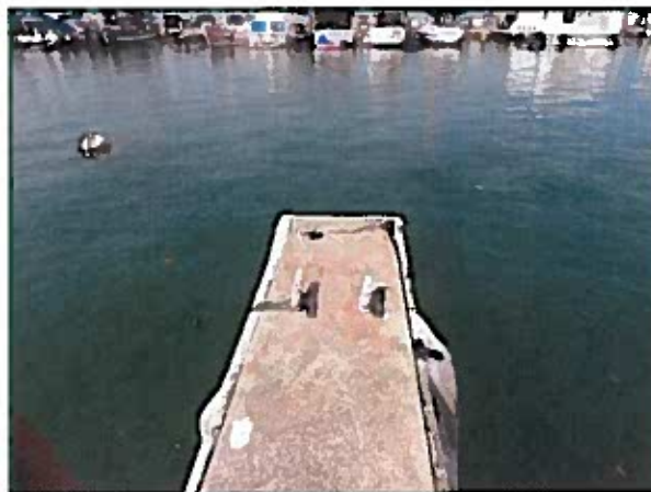
Representative view of an older fixed cement catwalk.
