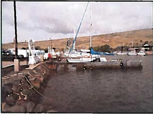
Representative view of catwalk moorings as seen from in front of the Harbor office looking west.
