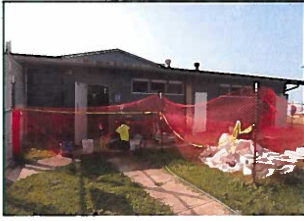
View of the private restrooms with showers, currently under construction.
