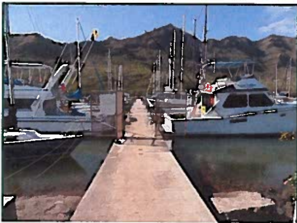
Typical Pier at Nawiliwili Harbor.
