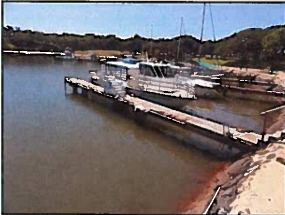
View of the harbor as seen from the northern most catwalk looking south toward the boat ramp.
