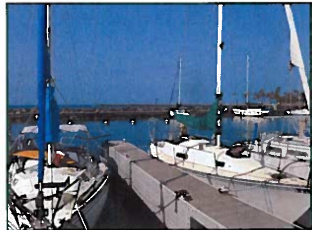
Representative view of a newer composite fixed catwalk.
