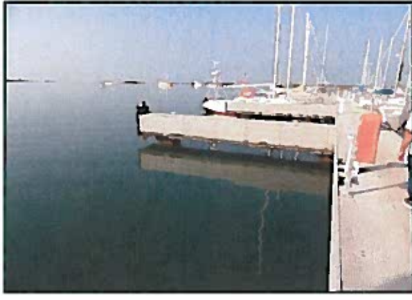
Representative view of a fixed dock made of composite material.
