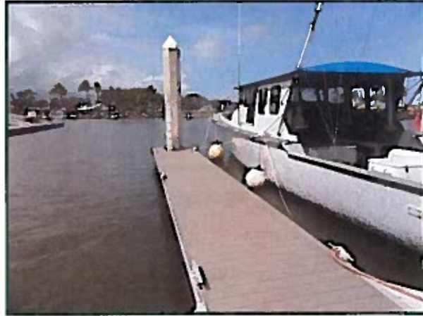
View of newer composite floating catwalk.
