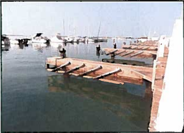
Representative view of fingers on fixed wooden pier.
