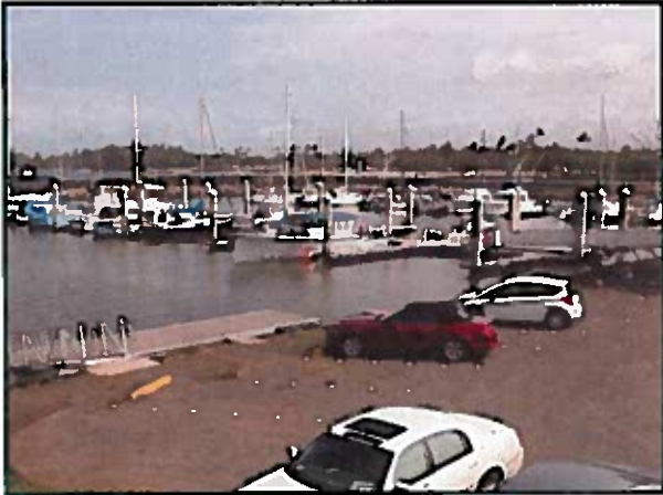
View of newly constructed floating pier 200, as seen from second floor of the Harbor office.
