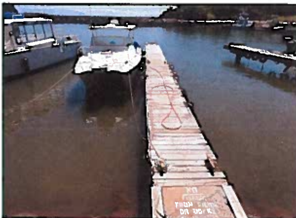
A wooden catwalk.
