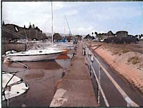
Tahiti moored vessels to a concrete pier.
