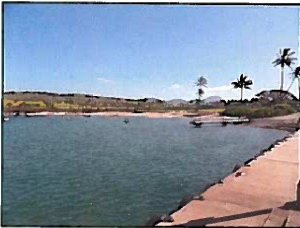
View of the boat ramp as seen from the loading dock.
