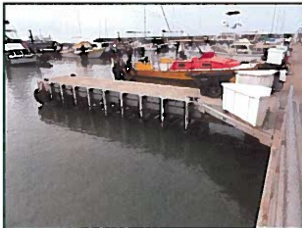
Representative view of catwalk with gear boxes on Pier C.
