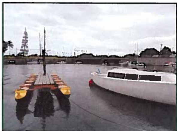
Southerly view of the outer basin at Wailoa Small Boat Harbor.
