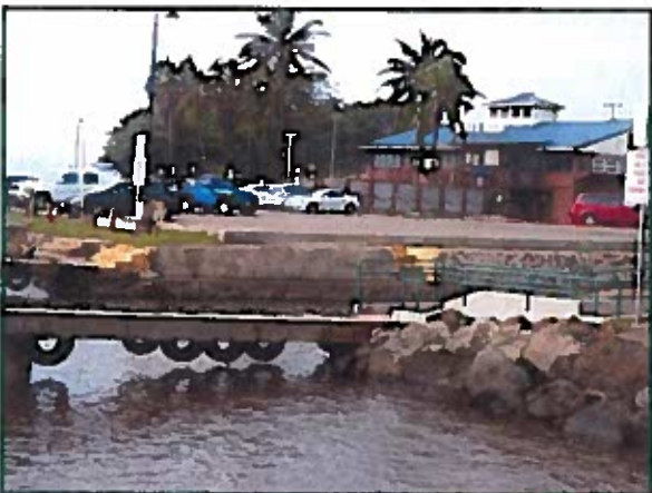
View of the loading dock and boat ramp in the background.
