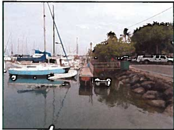
Older wooden fixed dock with Tahiti moorings.
