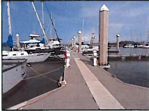
Newly constructed floating dock.
