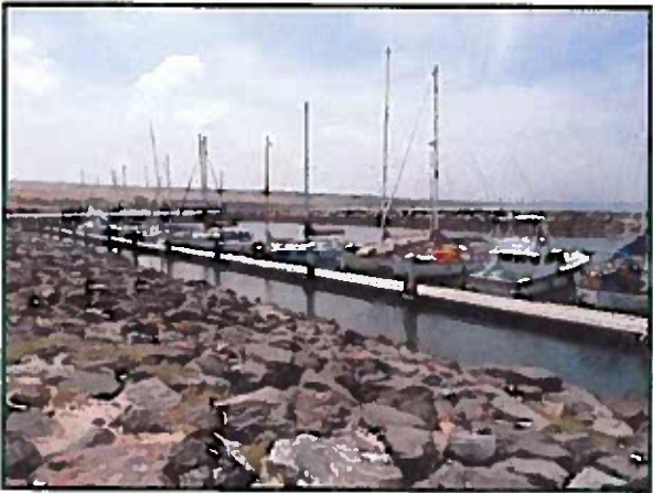
View of the newly constructed floating dock at South Kawaihae Small Boat Harbor.
