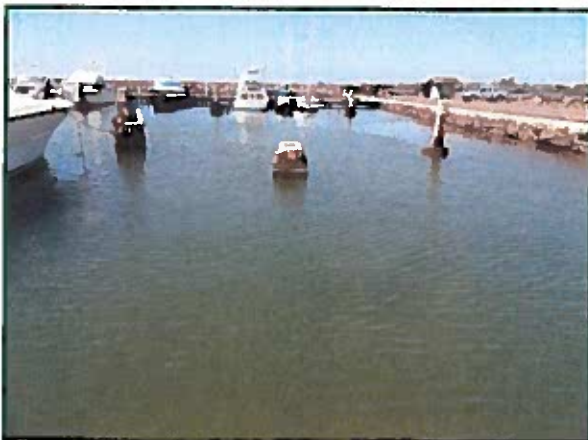
View of a collapsed catwalk.
