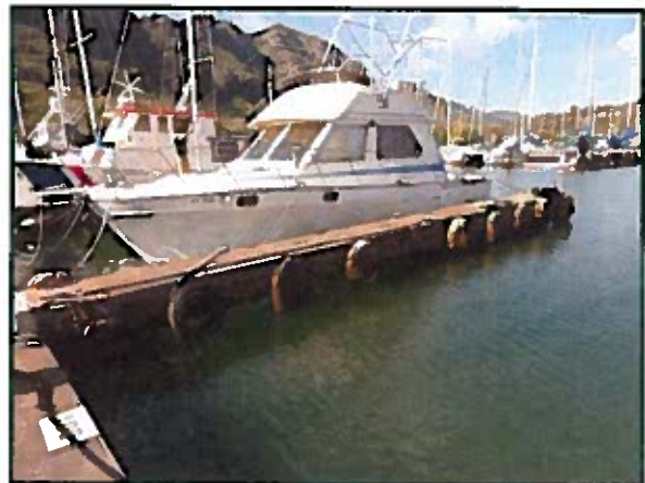
Typical catwalk mooring at Nawiliwili Harbor.
