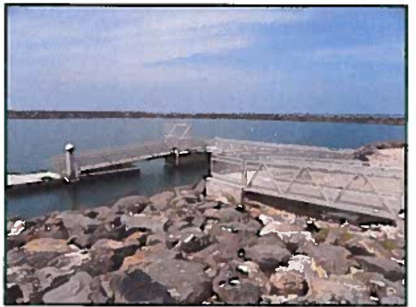
View of the access gate to the dock at South Kawaihae Small Boat Harbor.
