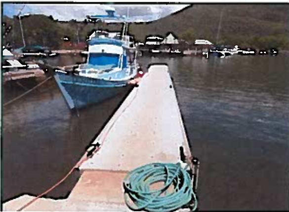
A fixed catwalk constructed of composite material.
