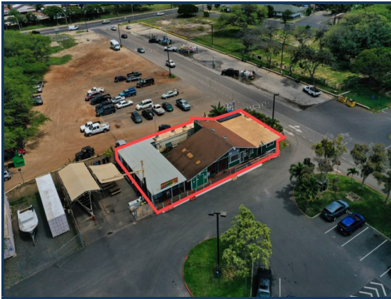
Drone aerial of subject outlined in red.
