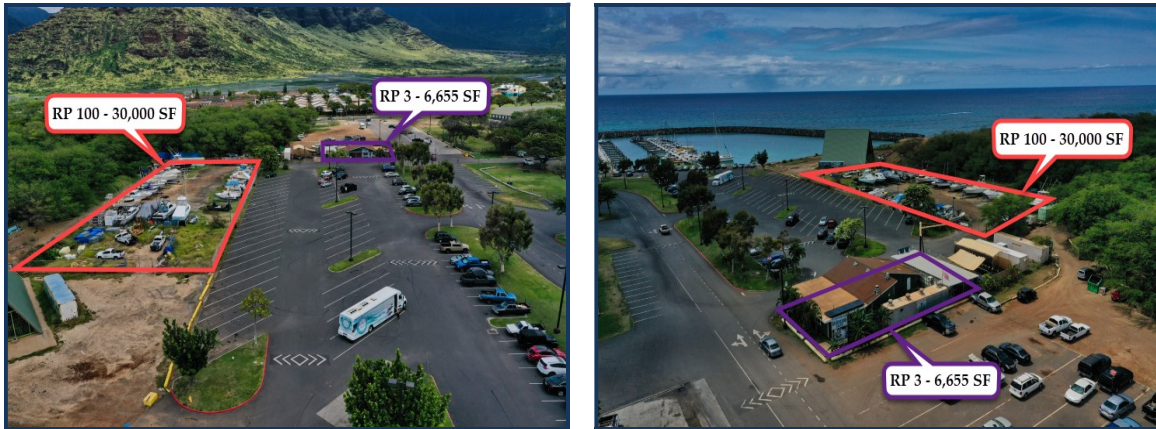
Drone aerial of subject RPs facing eastward (left) and westward (right).
