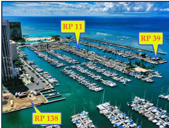
Harbor facing southeasterly.
