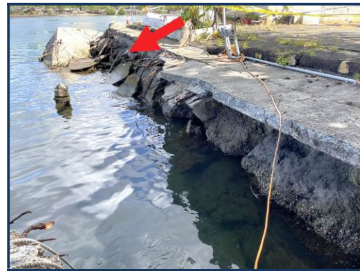
Annotated locations (red arrow) of the collapsed/lost portion of the makai pier (approx. 500 SF)
