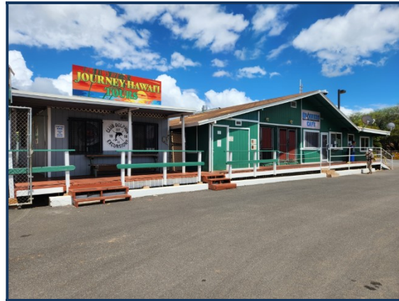
Permittee improvements on RP site.
