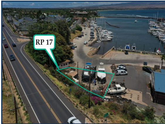
Aerial view of RP 17 facing northwest toward Maalaea Bay.
