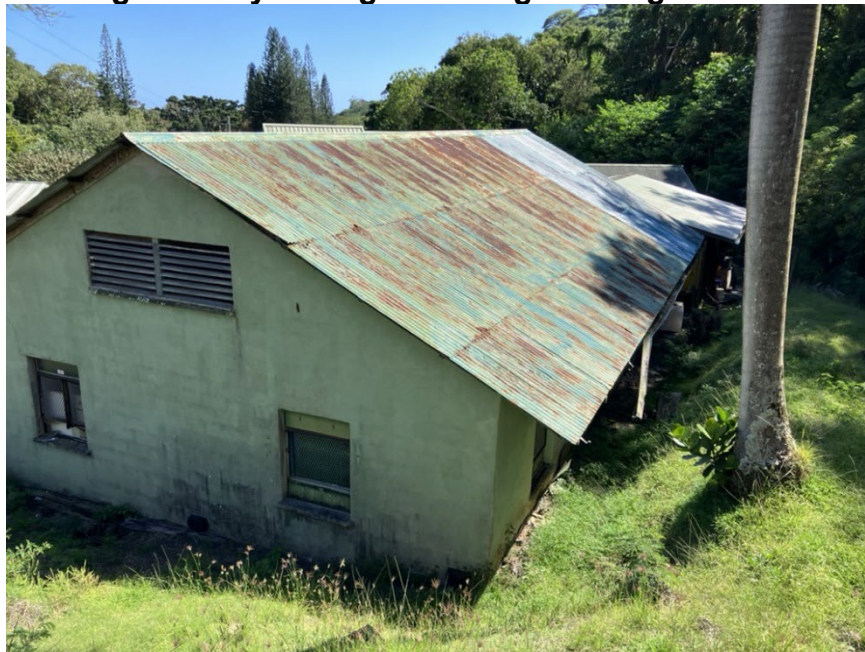
Figure 7. Existing Forestry Storage Building Looking South
