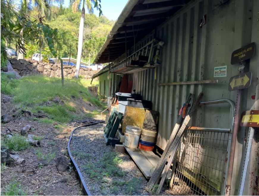
Figure 10. Rear of the Na Ala Hele and Forestry Storage Buildings Looking North
