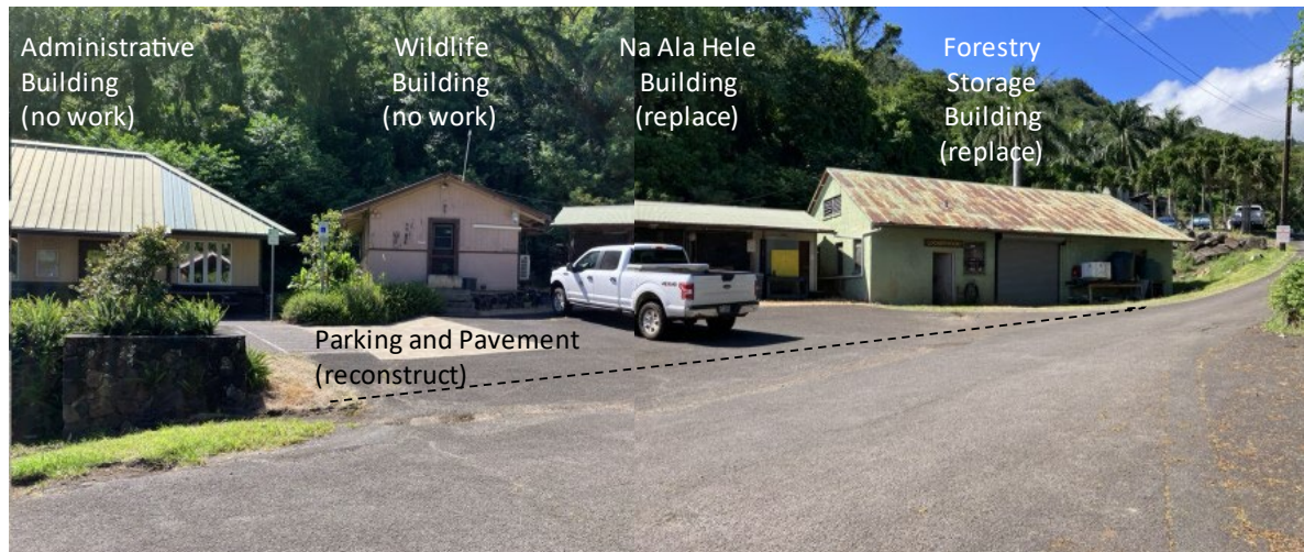
Figure 6. Existing Site Facing the Wildlife Building
