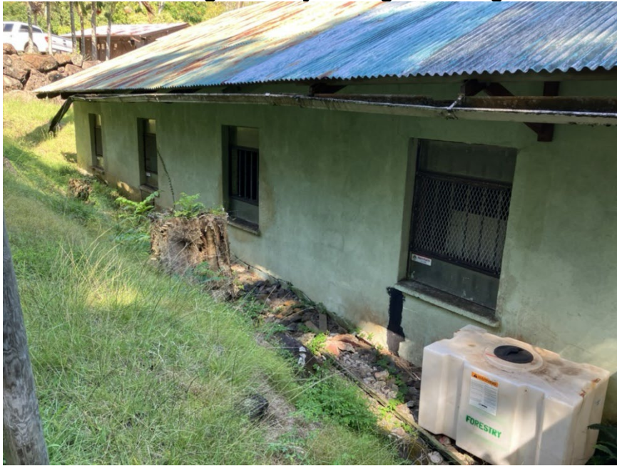
Figure 8. Rear of the Existing Forestry Storage Building
