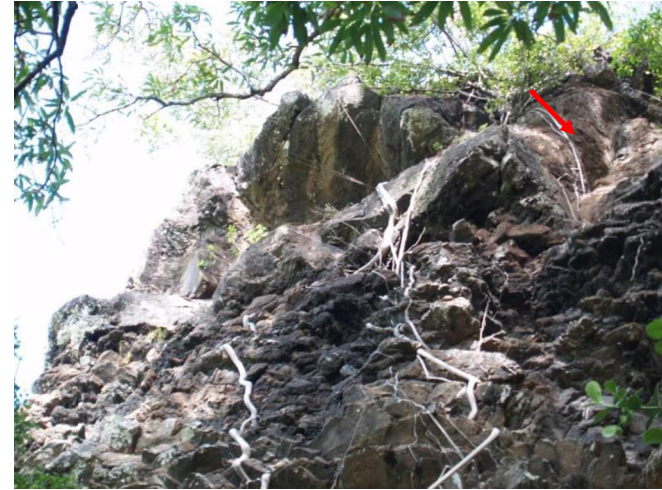
Photo 2-18. The source (pointed by the arrow) of the recent rockfall At B21.
