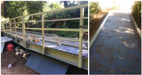
Examples of FRP path installation at McBryde Garden, Līhōʻi
