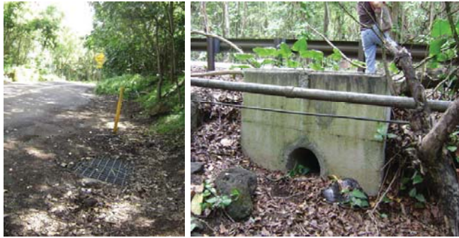
Figure 2: Typical Existing Drain Inlet along Kuhio Highway
