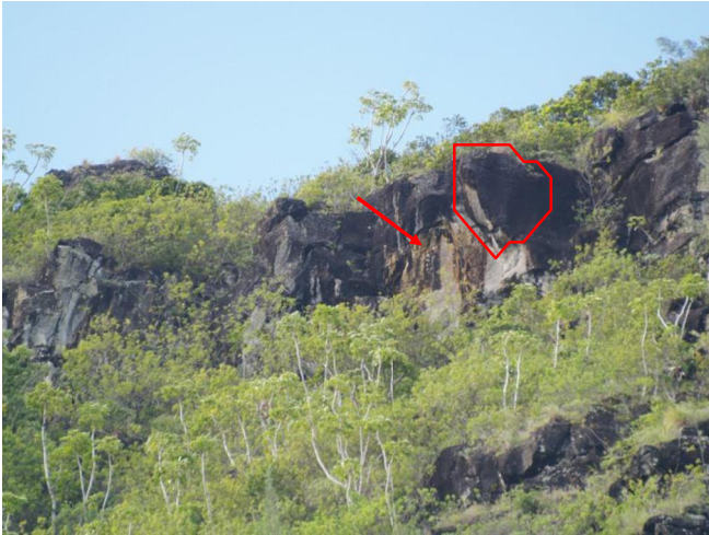
Photo 2-32. A recent rockfall source (pointed by the arrows) and a large overhanging rock with back fractures (indicated by the dashed lines) (photo taken from vantage point V2).
