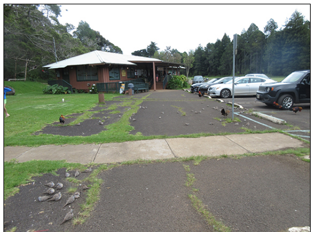
Asphalt pavement between Museum and Lodge.
