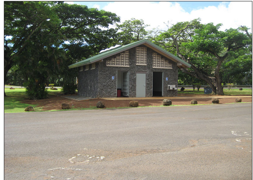
Detail of comfort station built in 2008 with wall-mounted water fountain.
