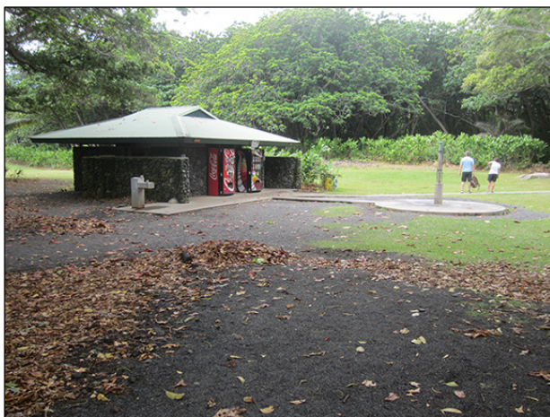
Comfort Station with water fountain and shower.
