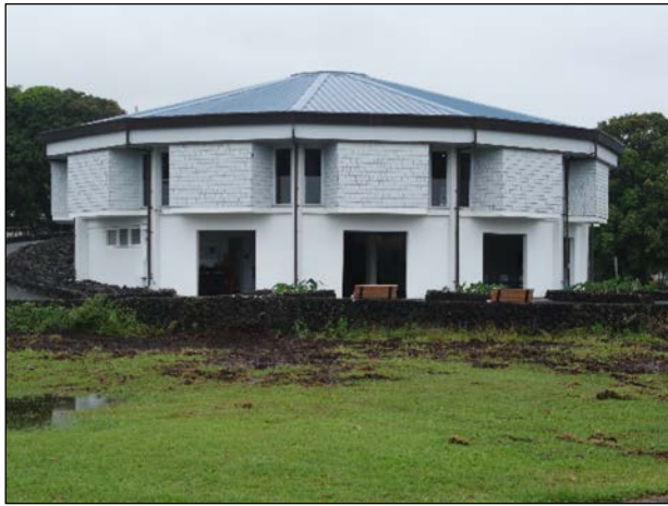
Framing of lānai doors on lower floor.
