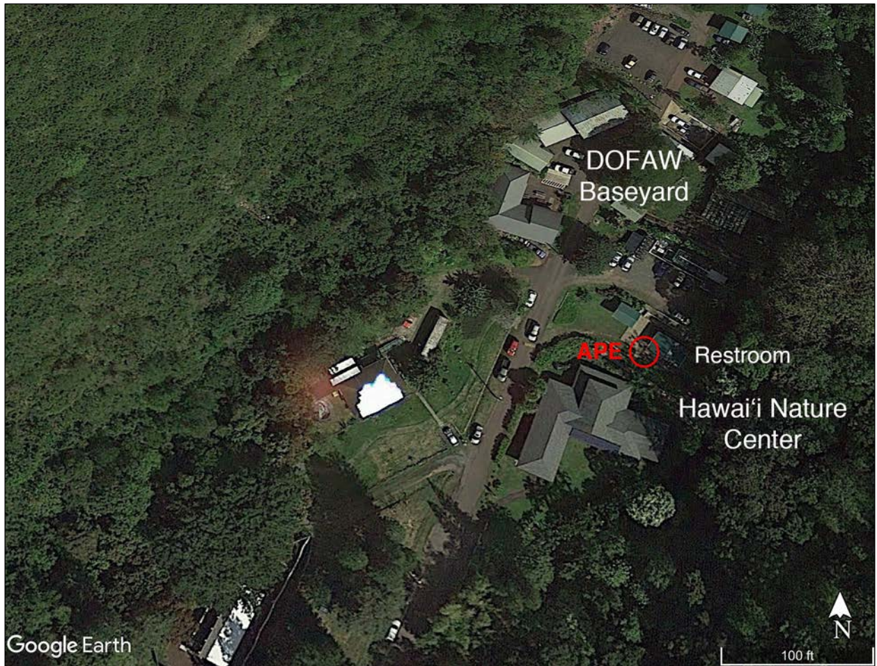
Fig. 41. APE at the Makiki restroom located between the Hawai'i Nature Center and the DOFAW Baseyard.
