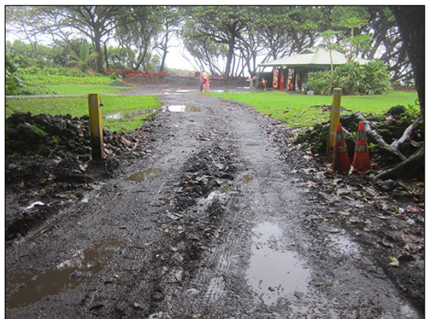
Service road through Site 5395, Feature A wall.
