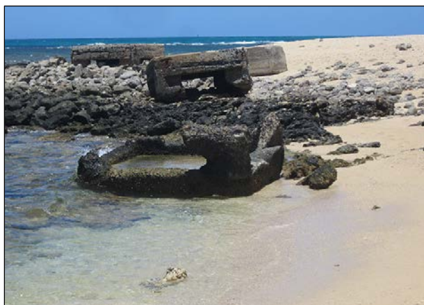
Site 6A: Remains of concrete pillboxes (1934-1943).
