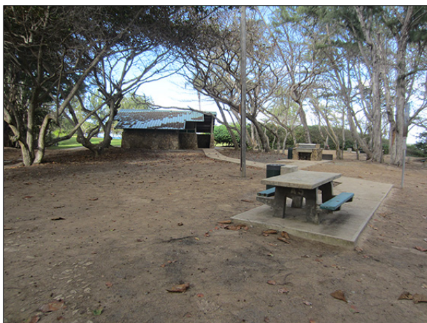
Comfort station within campground area A.
