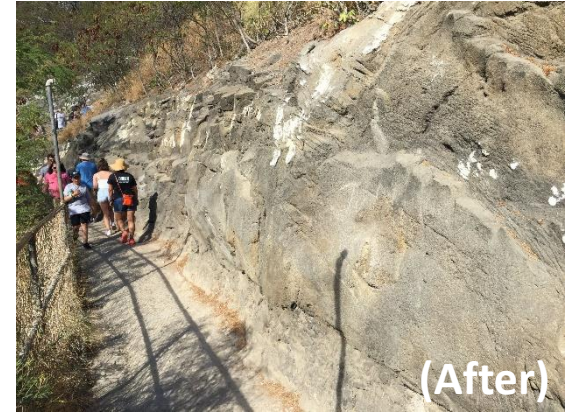
Proposed Shotcrete Example (Diamond Head Monument Rockfall Mitigation)
