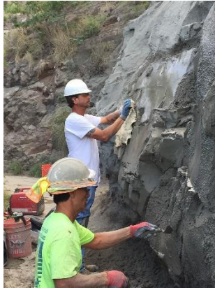
Proposed Shotcrete Example (Diamond Head Monument Rockfall Mitigation)
