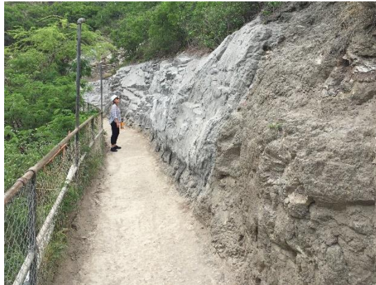
Proposed Shotcrete Example (Diamond Head Monument Rockfall Mitigation)
