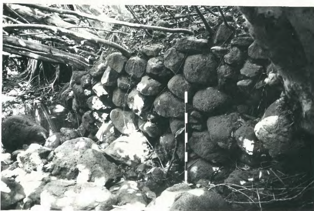
Figure 4. Part of the lower water diversion system, showing a section of cobble and boulder facing. Photo taken facing southeast.
