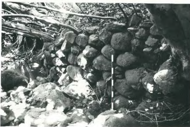
Figure 4. Part of the lower water diversion system, showing a section of cobble and boulder facing. Photo taken facing southeast.
