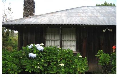
'Totong' (corrugated metal) was often installed over the remains of the original wood-shake roofing and purlins.
