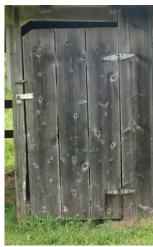
A variety of unpainted, rustic doors were built using vertical boards. Doors were sometimes used in pairs. Strap hinges were typical door hardware.
