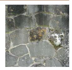
Mortar joints inappropriately sealed with caulk.
