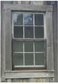
Above, these wood-framed double or single-hung windows are typical. The windows were used alone, or in pairs. and other multiple combinations.
