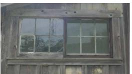
Six-light sash were typically used in sliding windows (above and left), although other muntin configurations are found (below).
