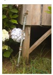
Apply environmentally safe chemical preservatives to wood features, including post ends at foundations, which are exposed to decay and are traditionally unpainted.
