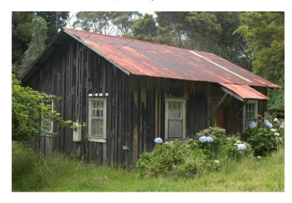
Historic buildings at Kōke'e generally retain their original roof form and detailing; however reroofing was often done with new materials, such as corrugated metal. Roofs have sometimes been adversely affected by the addition of new elements such as antennas, mechanical equipment, solar collectors, and satellite dishes.
