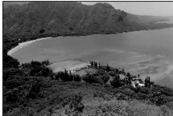
Huilua Fishpond in 1980 with wall damage.
