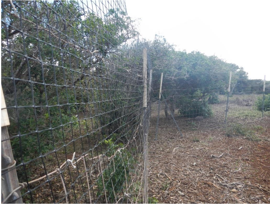
Figure 12. Retrofit to extend height of Lapaiki fence.
