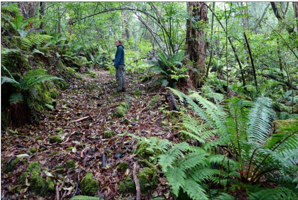
Figure 21: Upper Portion of Switchback. The trail grade was created by cutting the soil and rock embankment visible on the left and leveling what became the trail bed.
