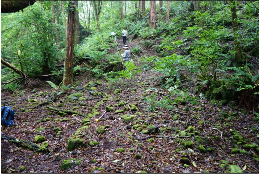
Figure 20: Trail Segment with Defined Curbstone Alignment. Beyond this segment is the start of a switchback that turns right after the incline visible in the photograph. An embankment cut defines the trail edge on the right hand side..
