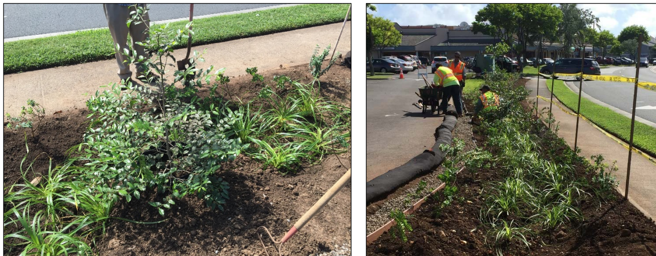
Figure 4.9. Raingardens being established as part of Kaulunani’s applied stormwater management project.
