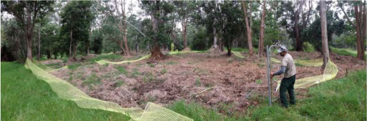
Figure 3. TMA staff constructing the temporary fence at the planting area.
