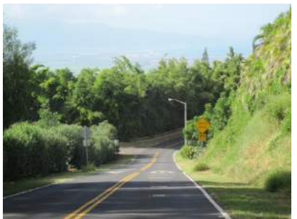
Heavy, hazardous unmanaged roadside fuels
