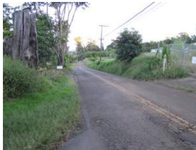
Hazardous roadside fuels on Makawao-Olinda Rd. near Seabury Hall
