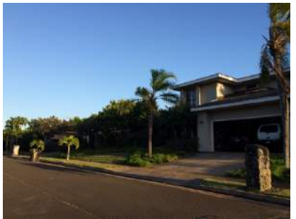
Example of tree hazard next to home windows
