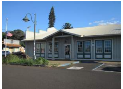
Hazardous fuels near post office
