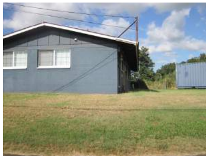
Kula Glen- example of maintained lawn and non-combustible siding
