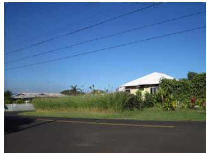
Example of home with hazardous fuels surrounding primary structure
