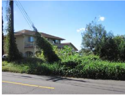
Hazardous vegetation growing on powerline
