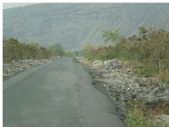
Photo 9. Green waste dumping along roadsides substantially increases fire hazard and likelihood of roadside ignition.
