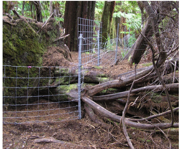
Figure 10: Example of ungulate fencing. Volcano, Hawai'i.
