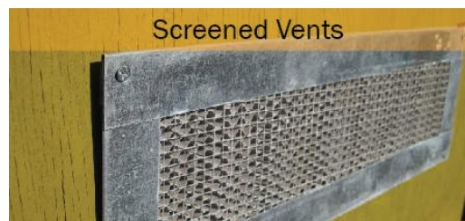
Figure 34. Covering vents with 1/8-inch or smaller metal mesh blocks embers from entering a home or structure.
