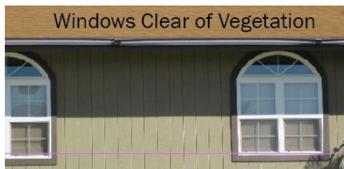
Figure 35. Keep windows free of vegetation to reduce likelihood of heat-caused breakage that lets embers into your home.
