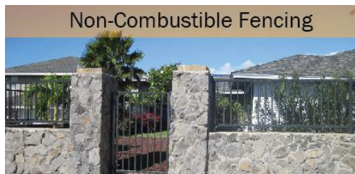
Figure 38. Wood fencing can act like a fire wick straight to a home. Use non-combustible materials for all fencing and yard structures.
