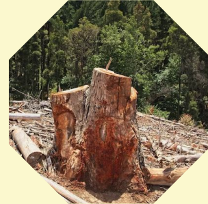
Land clearing, stump removal
