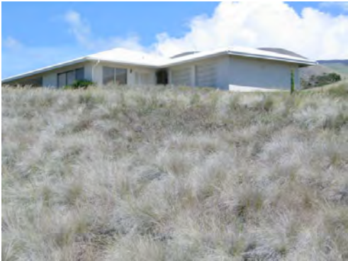
House in Kanehoa subdivision. Built atop a slight hill, the front yard is covered in invasive grasses, a potential wildfire hazard.
