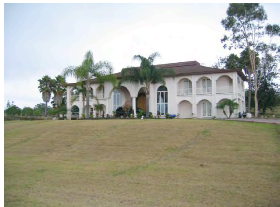
Typical house in Pu'u Lani Ranch Estates. This house has defensible space, although not all homes in the subdivision do.
