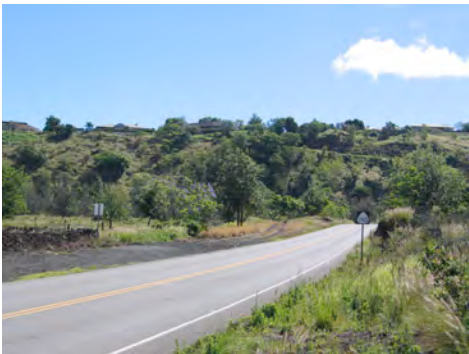
Ridge along the southern boundary of Pu'u Lani Ranch Estates subdivision. The ridge is a fire concern due to its steep slope and the high-intensity burning vegetation growing on the ridge.
