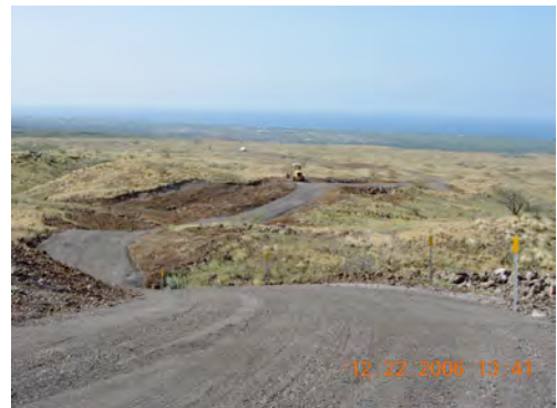
An emergency access road leading from Waikoloa Village to Queen Kaahumanu Highway was recently built to provide additional egress during wildfire emergencies.
