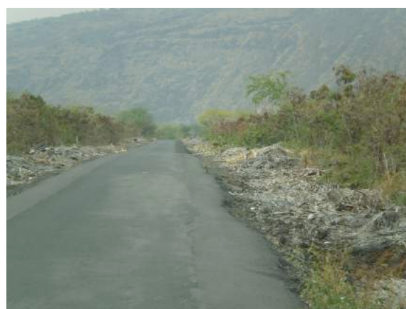
Photo 9. Green waste dumping along roadsides substantially increases fire hazard and likelihood of roadside ignition.
