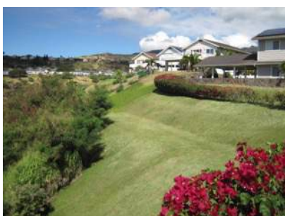
Fuelbreak on steep slope under homes in Pueonani neighborhood
