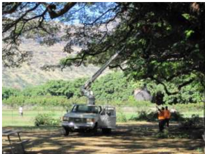
Active tree trimming at Pililaa Park
