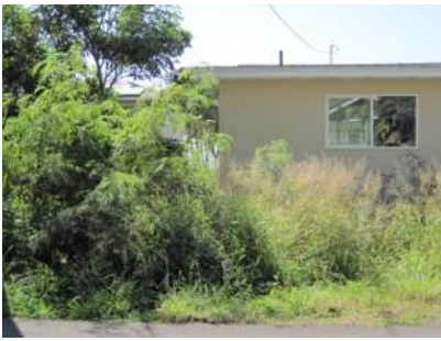
Overgrown vegetation next to one of a few abandoned homes
