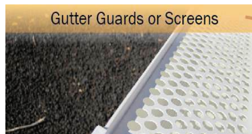
Figure 15. Rain gutters should have screens to keep leaf debris from accumulating. Maintain gutters to keep them clear and clean.
