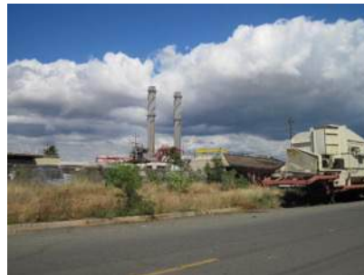
One of many areas in Industrial Park with unmanaged fuels along sidewalks
