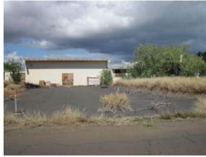
One of many abandoned buildings with unmanaged fuels near Kalaeloa Airport
