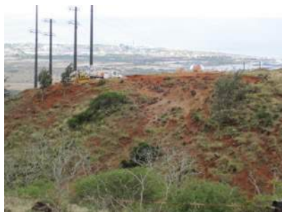
Example of heavy erosion
