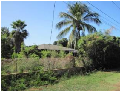
Home surrounded by flammable palms, shrubs, and grasses
