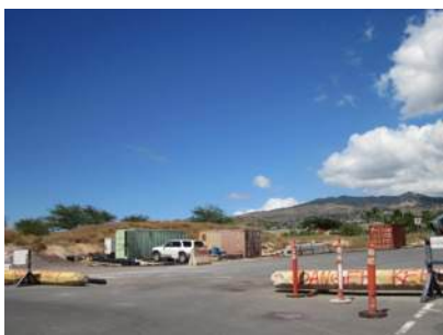
Construction for new Kekala Street development with pockets of unmanaged vegetation
