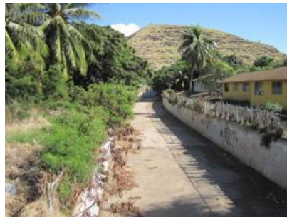
Homes along canal off of Plantation Road across from overgrown wildland
