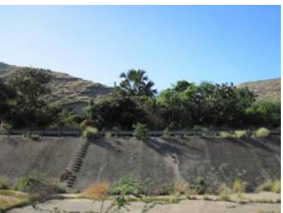
Homes along the canal with dense fuels surrounding them
