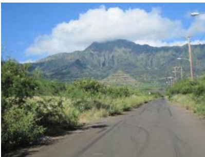
Kolealiilii Street an ignition hazard with tall grass and ‘ekoa on shoulders and ATV traffic
