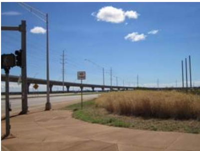
Small fuelbreak cleared alongside sidewalk on Kualaka'i Parkway
