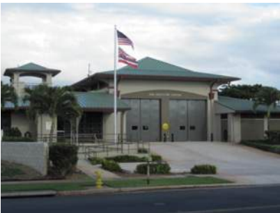
‘Ewa Beach Fire Station
