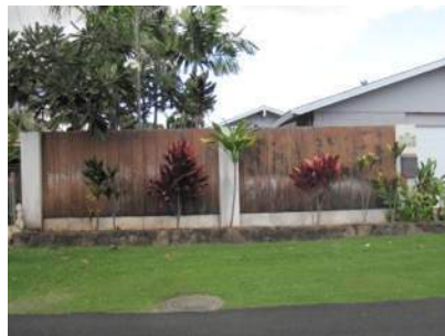
‘Ewa Beach Road home with fire-free zone along combustible fence line
