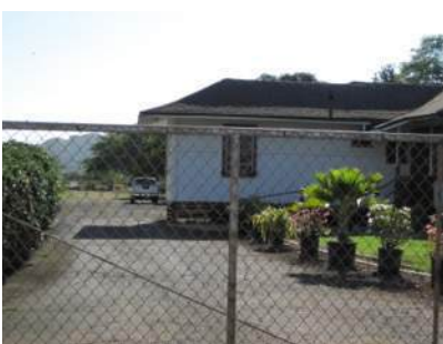
Example of good defensible space and fire-free zone
