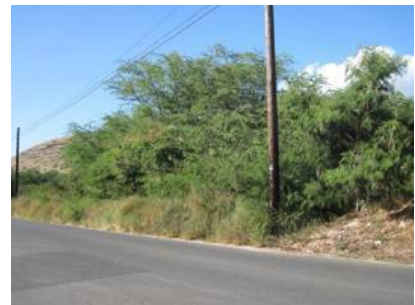
Example of roads with no vegetation management on shoulders under powerlines
