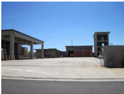
East Kapolei Fire Station
