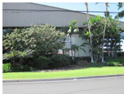
Example of good defensible space around Industrial Park building
