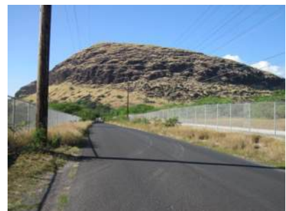
Paakea Road with shoulders overgrown with grasses and 'ekoa
