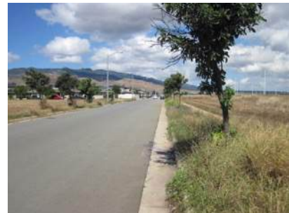
Dry grass on sidewalk along Kekahili Street
