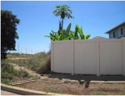
Dry grass growing up onto combustible fence near home
