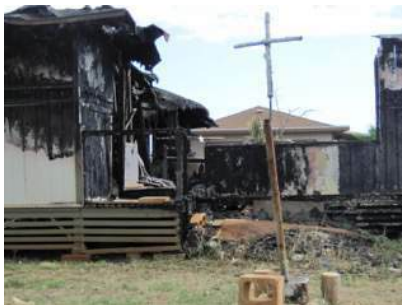
House on Peone Place that burned down in structure fire
