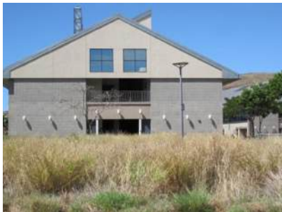
UH West O'ahu building adjacent to area of flammable unmanaged grass
