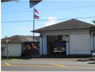
Kalaheo Fire Station
