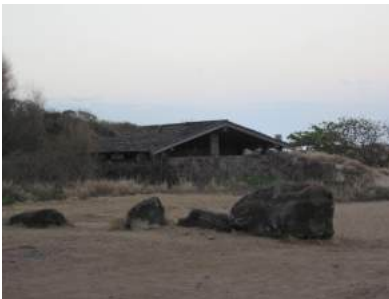
Polihale restroom facilities surrounded by fuels
