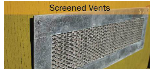
Figure 11. Covering vents with 1/8-inch or smaller metal mesh blocks embers from entering a home or structure.
