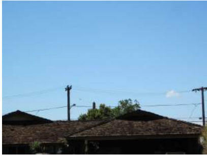
Example of shake roofs
