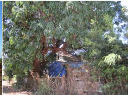
Overgrown vegetation along and over home
