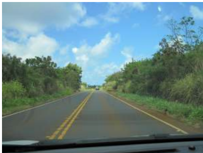
No shoulders along Olohena Road
