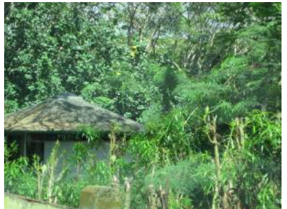
Makai side home in gulch surrounded by tall trees and with debris on roof
