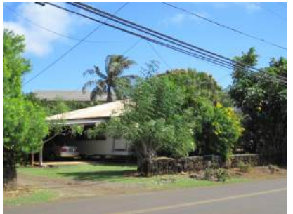
Typical home in area – good defensible space
