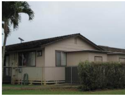
Common shingle roofs and wood sidings in Umi Street neighborhood
