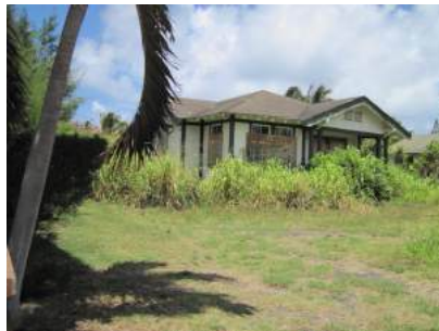
Vacant home with tall grasses surrounding structure
