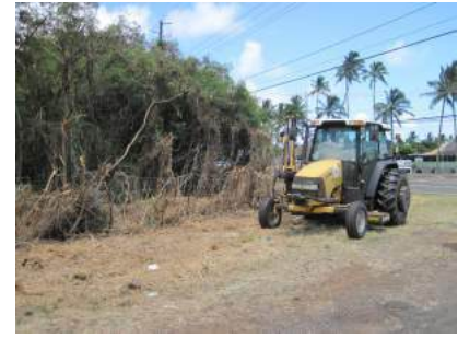
Area being cleared along busy intersection off of Kuhio Highway
