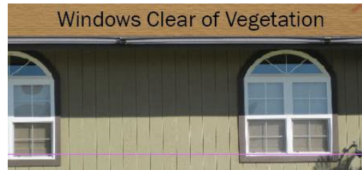
Figure 12. Keep windows free of vegetation to reduce likelihood of heat-caused breakage that lets embers into your home.
