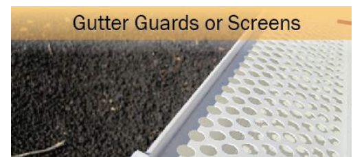
Figure 14. Rain gutters should have screens to keep leaf debris from accumulating. Maintain gutters to keep them clear and clean.
