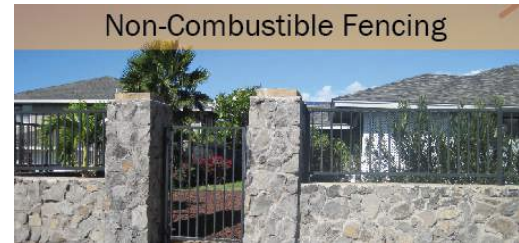
Figure 15. Wood fencing can act like a fire wick straight to a home. Use non-combustible materials for all fencing and yard structures.
