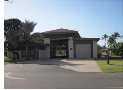
Kihei Fire Station
