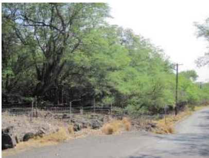
Vegetation overgrowing powerlines is a high hazard
