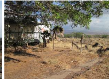
Abandoned lot with unmanaged vegetation
