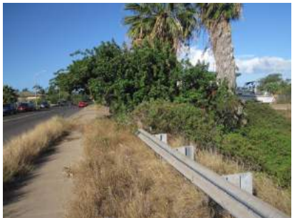
Roadside fuels on Halehuai Street
