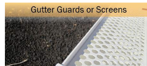
Figure 9. Rain gutters should have screens to keep leaf debris from accumulating. Maintain gutters to keep them clear and clean.
