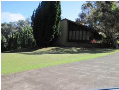
Example of property with good defensible space
