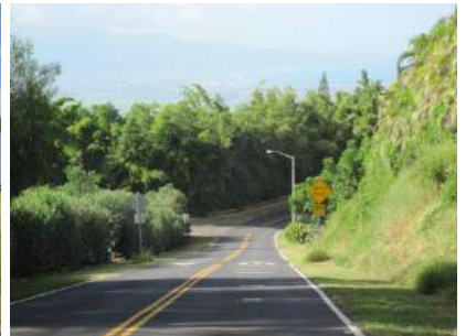
Heavy, hazardous unmanaged roadside fuels
