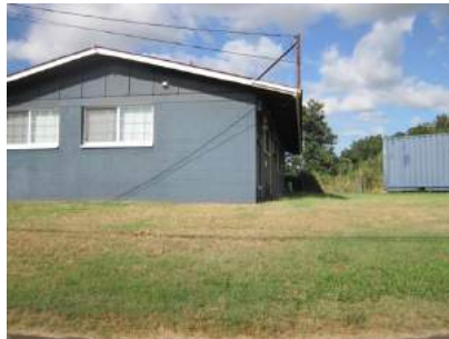
Kula Glen- example of maintained lawn and non-combustible siding
