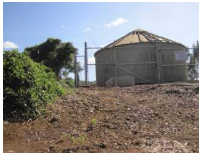
Kealakupu Drive water tank
