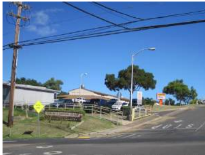
Pukalani Elementary School
