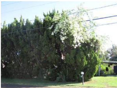
Vegetation overgrowing powerlines is a high hazard
