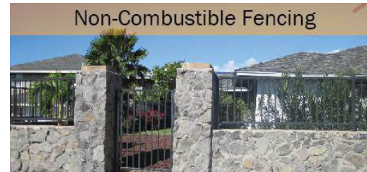
Figure 16. Wood fencing can act like a fire wick straight to a home. Use non-combustible materials for all fencing and yard structures.
