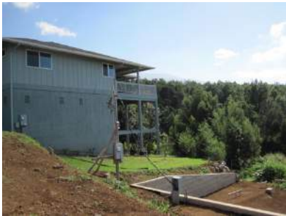
Example of home along wildland boundary
