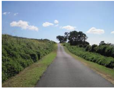
Kealakupu Drive paved road with cleared shoulders
