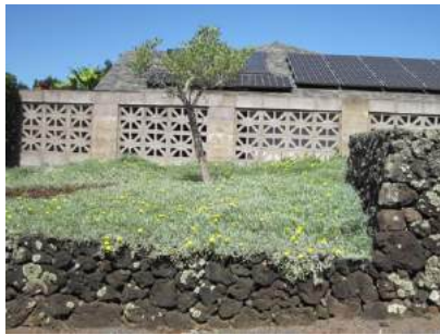
Good example of using groundcovers along edge of road and non combustible fencing/roof
