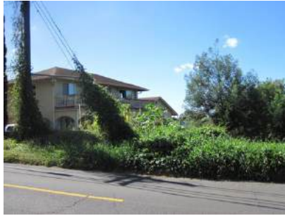
Hazardous vegetation growing on powerline
