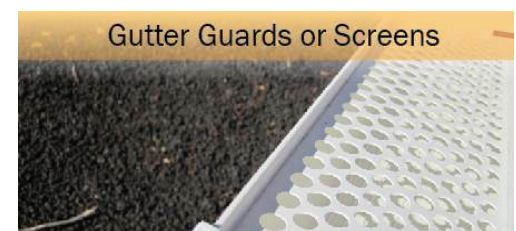
Figure 15. Rain gutters should have screens to keep leaf debris from accumulating. Maintain gutters to keep them clear and clean.
