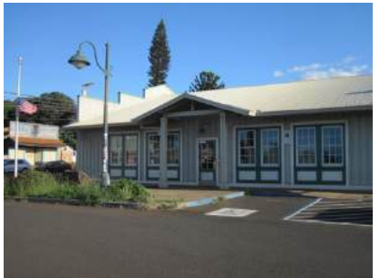
Hazardous fuels near post office
