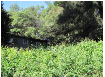
Example of heavy buildup of fuel around and over home
