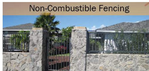
Figure 38. Wood fencing can act like a fire wick straight to a home. Use non-combustible materials for all fencing and yard structures.
