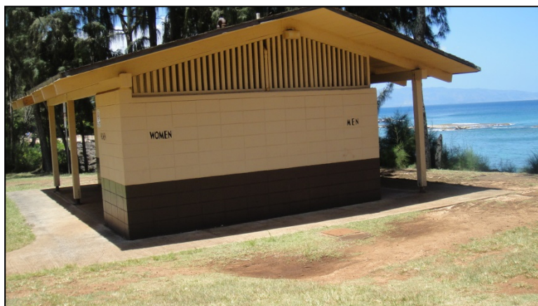
Comfort stations require maintenance to keep up with heavy use.
