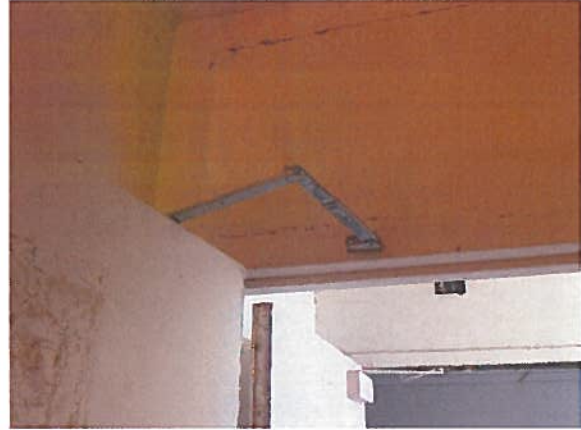
Ensure all self closing hardware on property is properly installed
