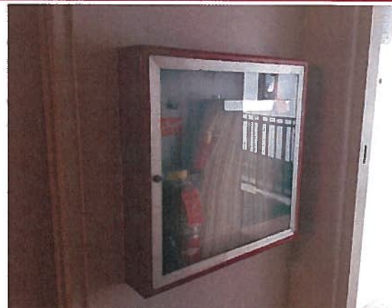
Fire extinguisher and hoses are not accessible, as glass does not have tool to break glass available
