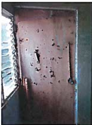
Exit door with major termite damage.
