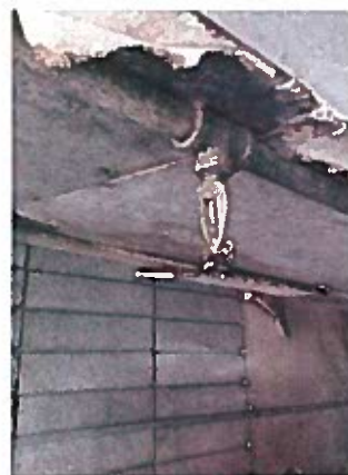
Fire sprinkler heads in trash enclosure with physical damage.
