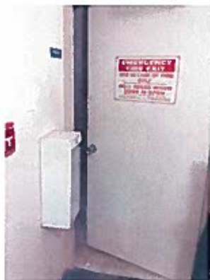
Fire extinguisher box obstructing exit door.
