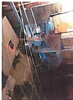
Electrical room with opening to upper floor water leaks onto electrical equipment.
