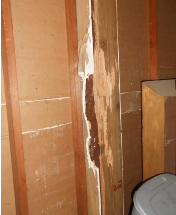
Photo 9: DSCN0487 – Termite damage in wood column in Electrical Room
