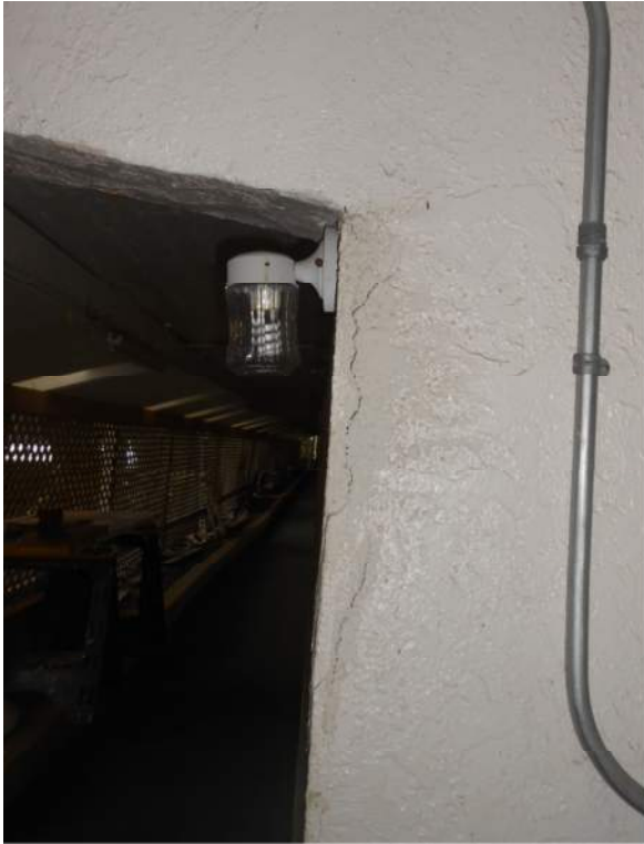
Photo 5: DSCN04888 – Crack with delamination at wall in Kitchen Wing
