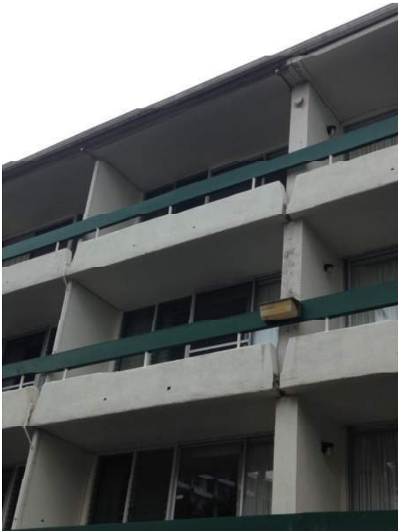
Photo 15: IMG_2552 – Area with exposed hollow core plank edges
