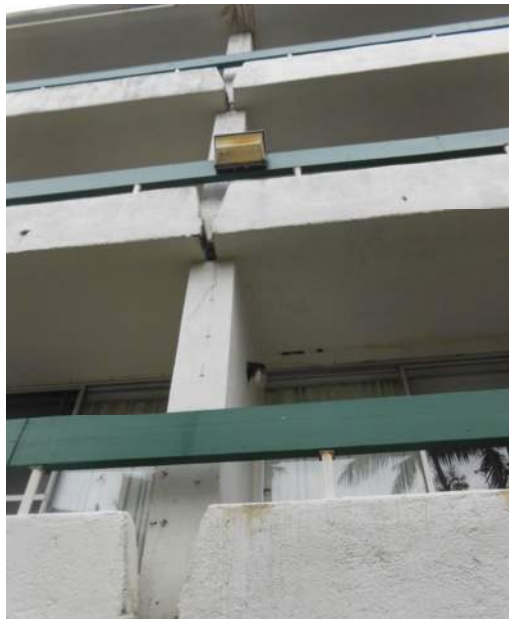
Photo 8: DSCN0501 – Cracking at Exterior Balcony Wall
