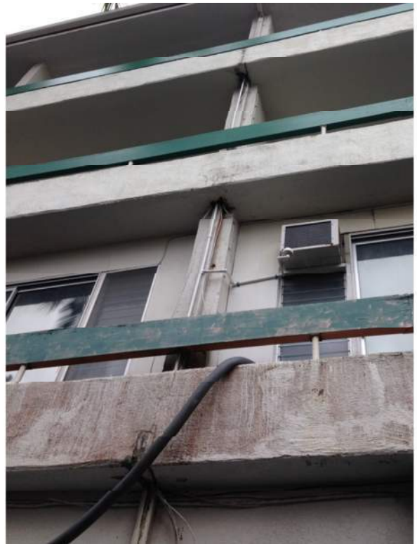
Photo 16: IMG_2555 – Deteriorating timber railing and balcony cracking
