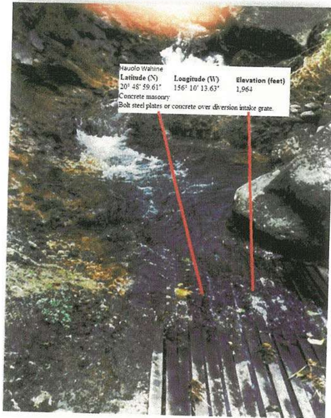
Photo 9 (above): Hauolowahine at Hauolo Ditch; intake at Hauolowahine Stream, tributary to Palauhulu Stream (K-30)
