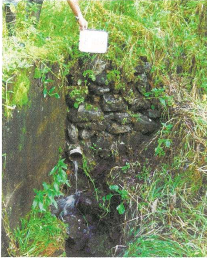
Photo 15 (above): Eight-inch (steel) pipe intake east of #9 (intake) (K-21a)
