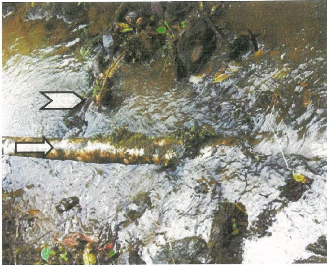
Photo 13 (above): Three-inch (aluminum) pipe intake by #6 control house at Koolau Ditch (K-19a) Photo 14 (below): Wailuanui #8 intake at Koolau Ditch (K-20a)
