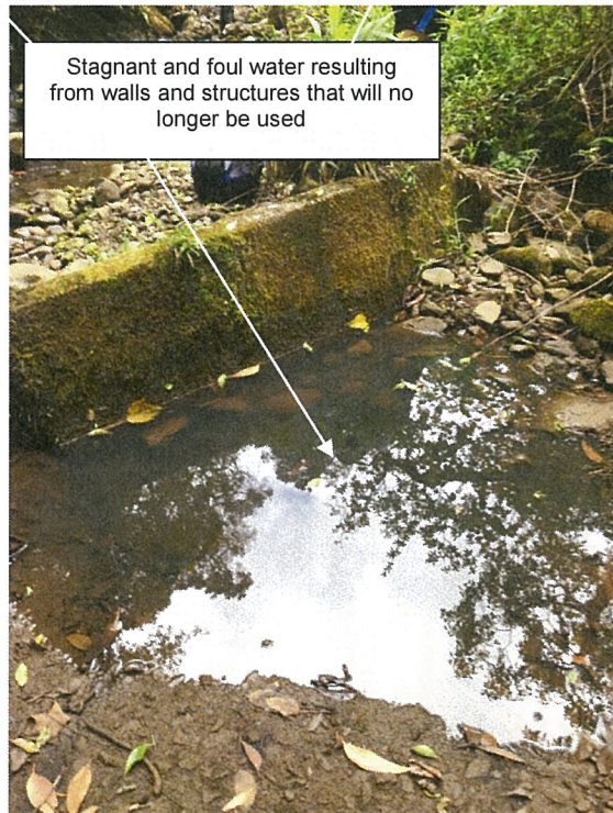
Figure 4. Stagnant water standing in depressions created by the walls and the gate structure.
