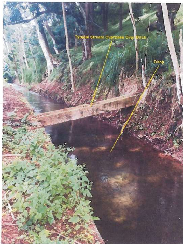
Photo 6 (below): Typical “stream overpass” intended to prevent the ditch from intercepting a stream
