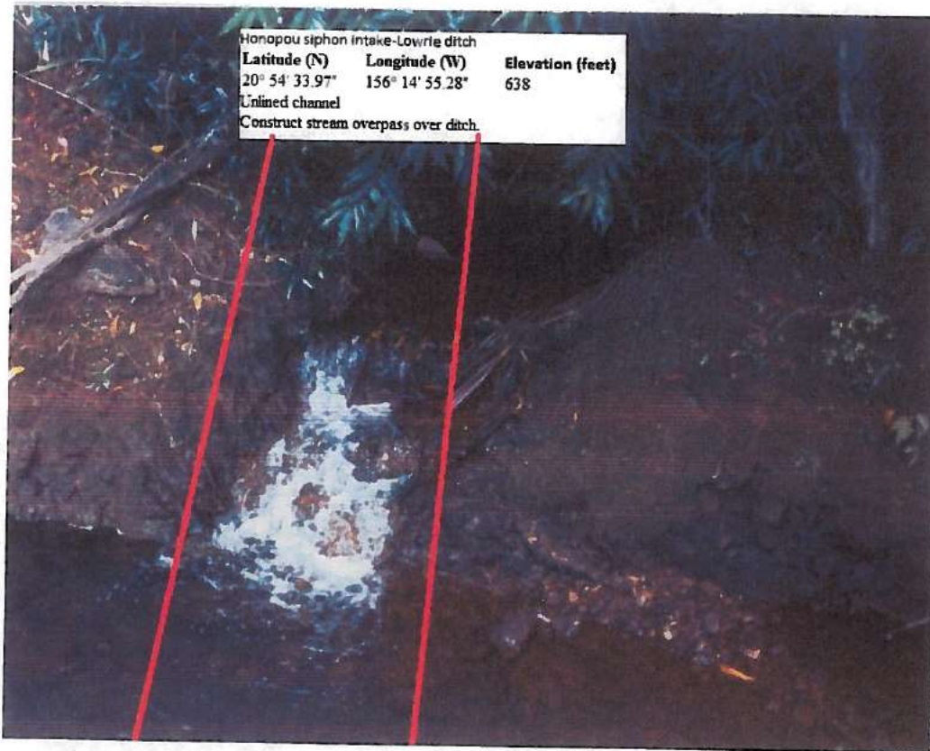
Photo 3 (above): Honopou siphon at Lowrie Ditch (L-16)
