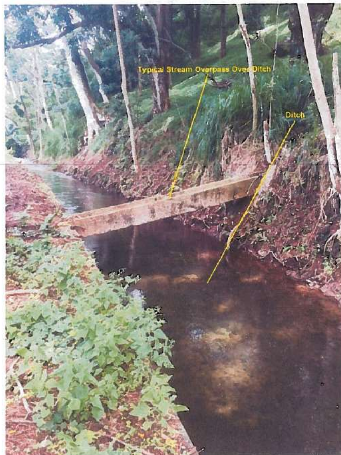
Photo 1 (above): Honopou long strainer at Lowrie Ditch (L-15) Photo 2 (below): Typical “stream overpass” intended to prevent the ditch from intercepting a stream
