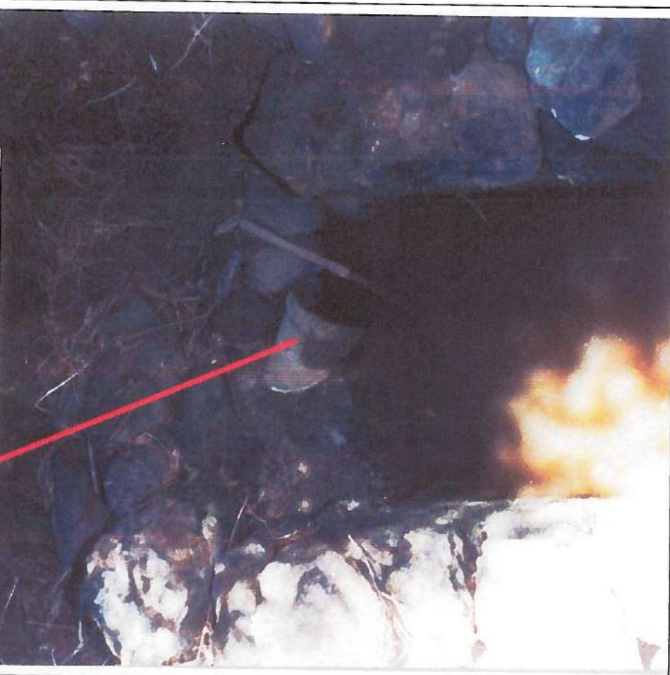
Photo 2: 6-inch Kualani (East Waiokamilo) aluminum pipe at Koolau Ditch (K-22a) Pipe shown was removed in 2007.
