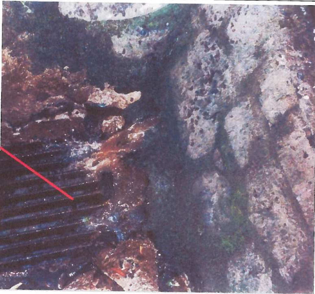
Photo 1: East Waiokamilo (Kualani) at Koolau Ditch (K-22/326.6) Diversion intake grate shown was sealed with concrete in 2007. (Note: Orientation of photo from 2008 IFSAR for Waiokamilo Hydrologic Unit appears incorrect; rotate counter-clockwise 90 degrees.)
