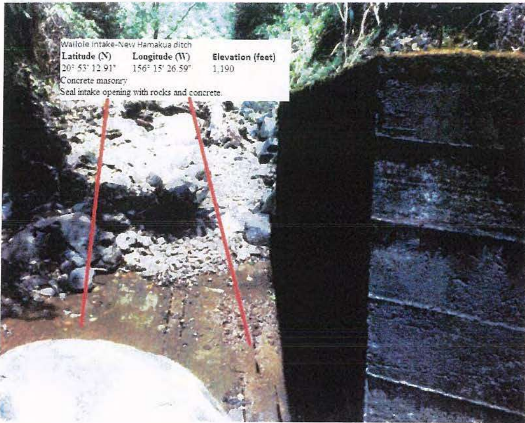
Photo 3 (above): Wailole at New Hamakua Ditch (NH-23)
