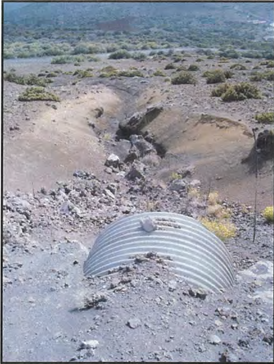
Figure 3-11. Mid Mountain Drainage Infrastructure
