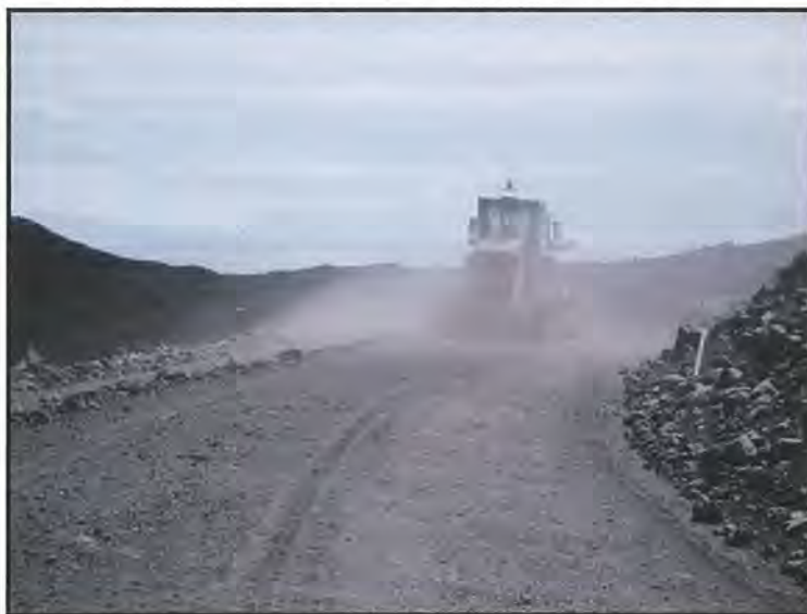
Figure 3-10. Road Grading on Mauna Kea Summit Access Road
