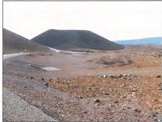
Batch Plant Staging Area
