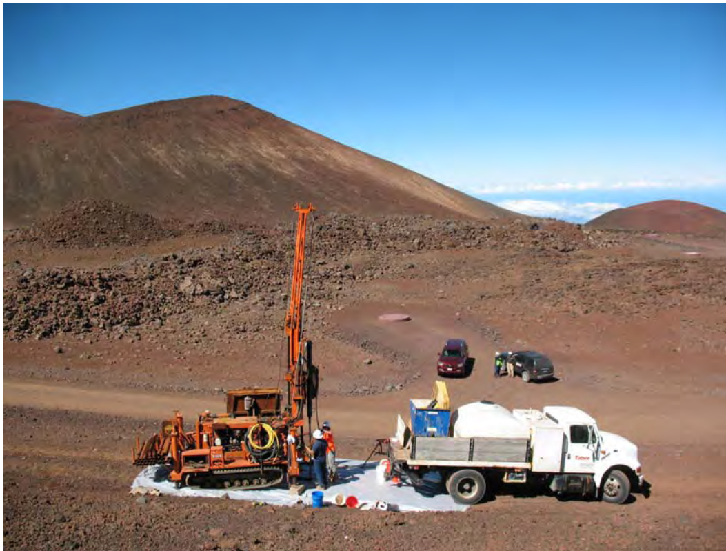
Figure 9. CME 55 HD crawler drill rig.
