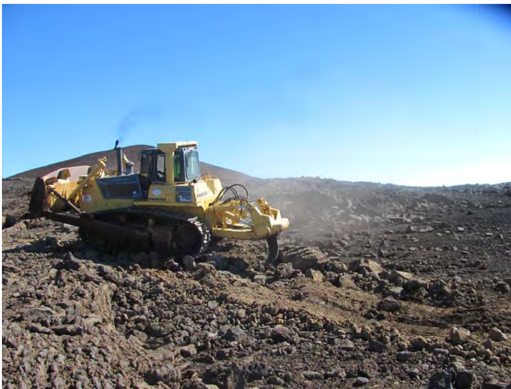
Figure 8. Komatsu 275AX bulldozer ripping existing 4WD road, Pu'u Pohaku in background.
