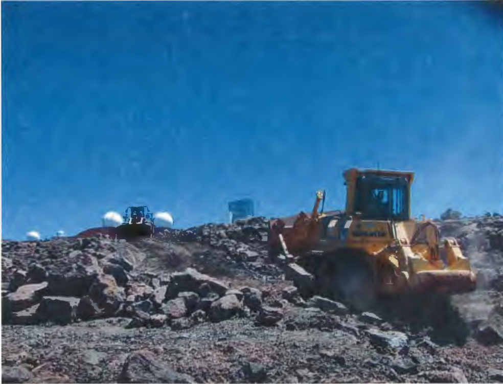
Figure 7. Komatsu 275AX bulldozer and Komatsu WA500 loader grading the existing 4WD road, note observatories in background.
