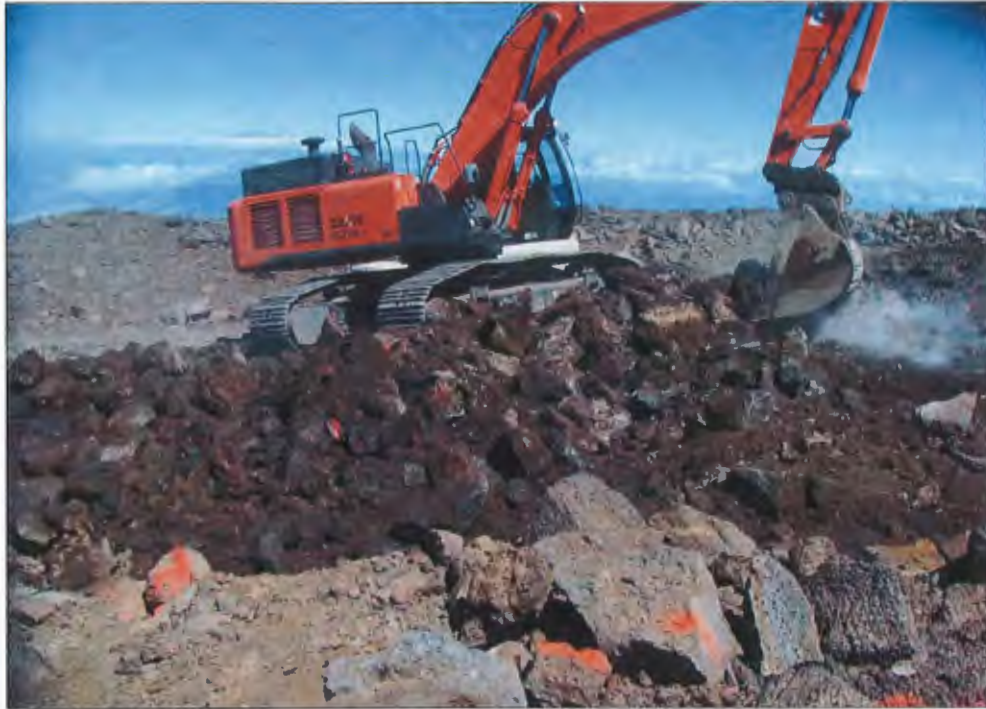
Figure 9. Hitachi 470 Excavator cutting eastern slope of groundbreaking ceremonial site pad.
