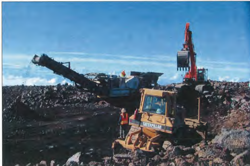
Figure 10. Groundbreaking pad excavated and partially graded.
