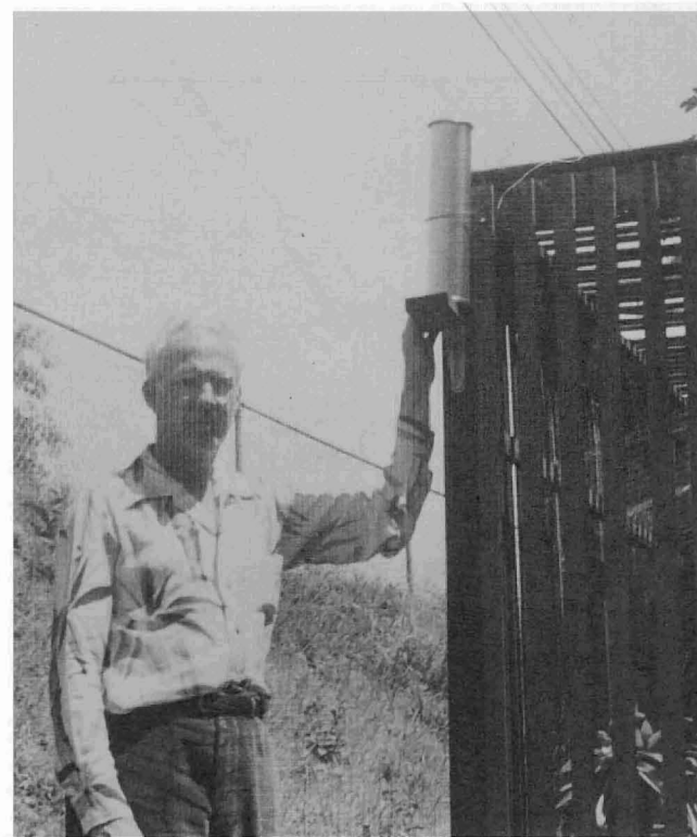
Standard 3-inch metal reduction tube also requires use of dip stick for measurement.
