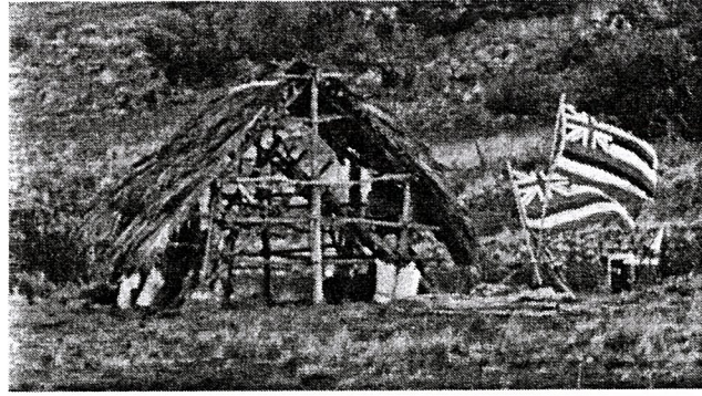
Figure 1: Protestor "Hale" in process of being built with 'ōhi'a wood and non-native palm fronds.
