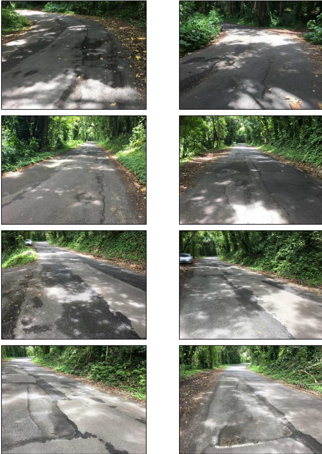
Figure 3.6 Existing Conditions in the Vicinity of 3300 Block of Tantalus Drive
