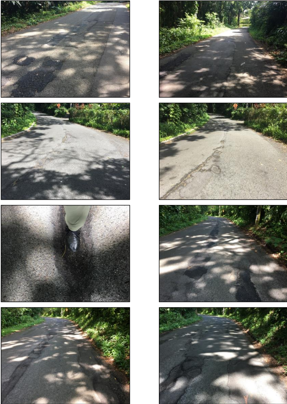
Figure 3.5 Existing Conditions in the Vicinity of 3700 Block of Round Top Drive
