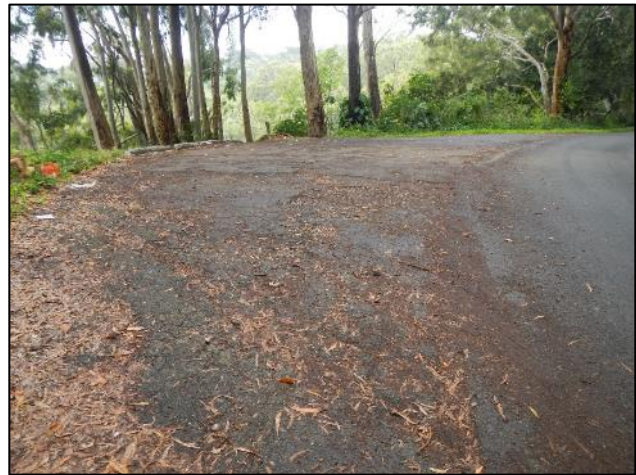
Uphill view of area T6.
