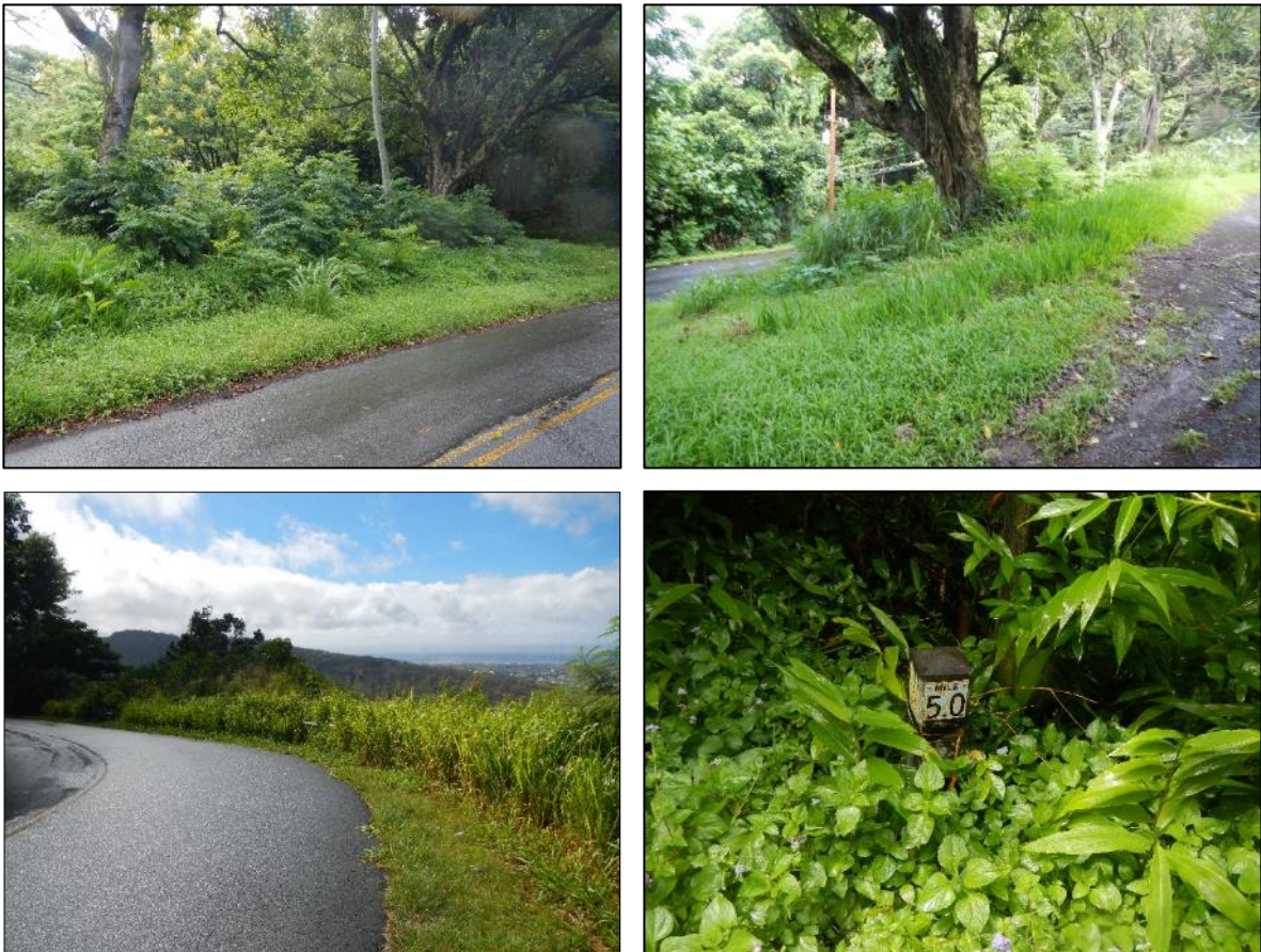
Figure 4.6 Examples of Vegetation Impacting Road Visibility
