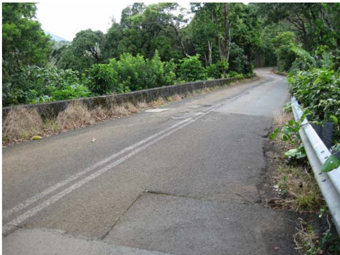
Figures 17 and 18: “Hogsback”, near Mile Marker 4.0 Basalt (lava rock) retaining wall at Hogsback.
