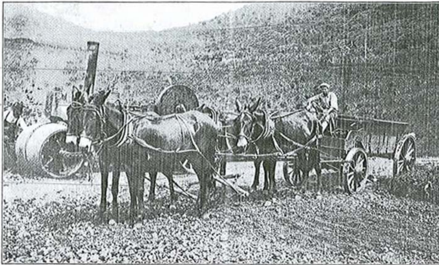
Figures 11 and 12: Paving Round Top Road, ca. 1916 ( Hawaii State Archives ) Paving Round Top Drive, ca. 1926 ( Williams Studios, Hawaii State Archives )
