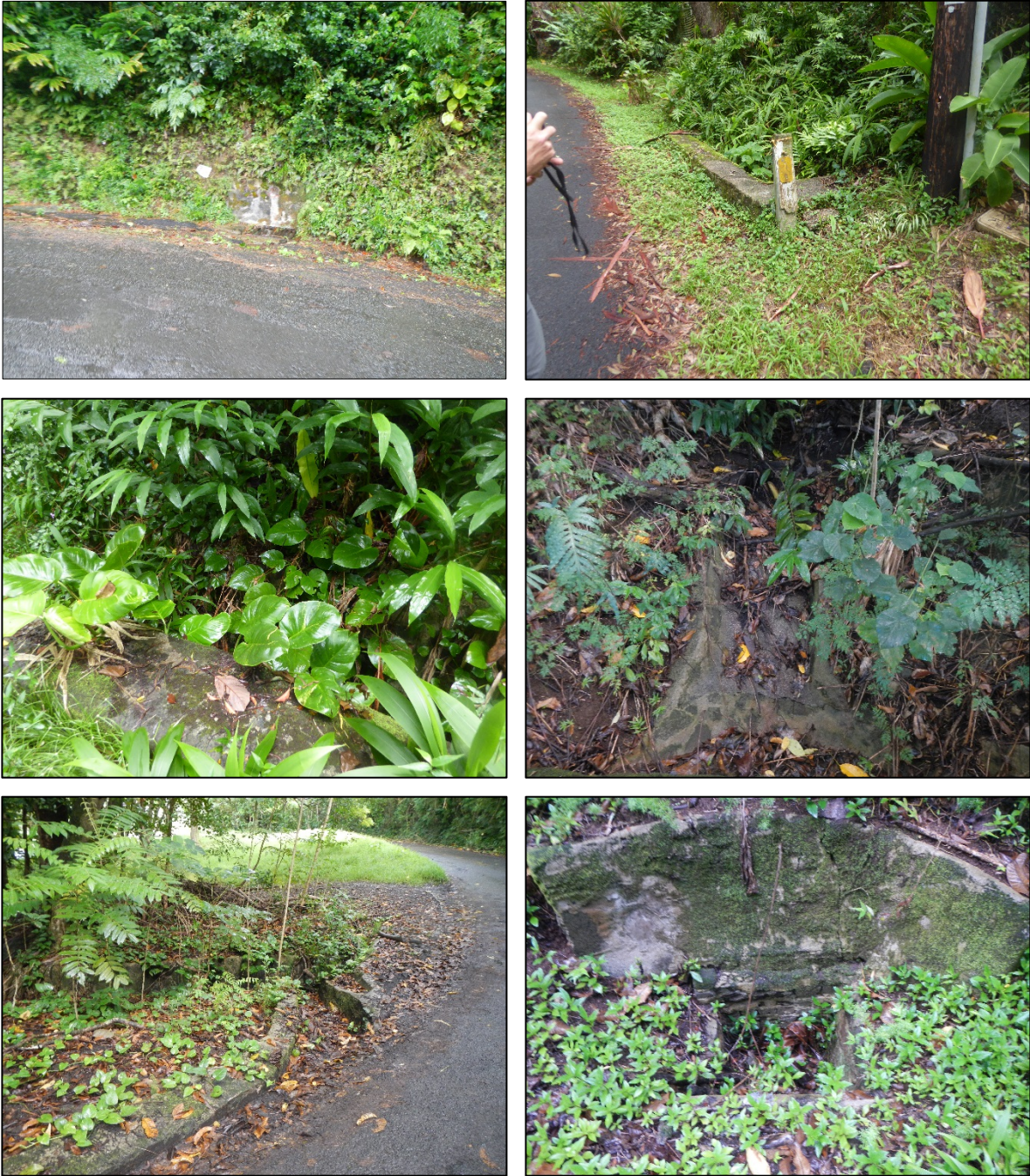
Figure 3.21 Typical Drainage Structures Along the TRTD Corridor
