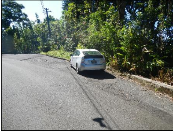
Paved parking area T12 on makai side of road.
