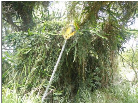
Sign obscured by vegetation
