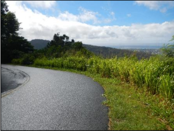
Tall grass has completely obscured the guardrail.
