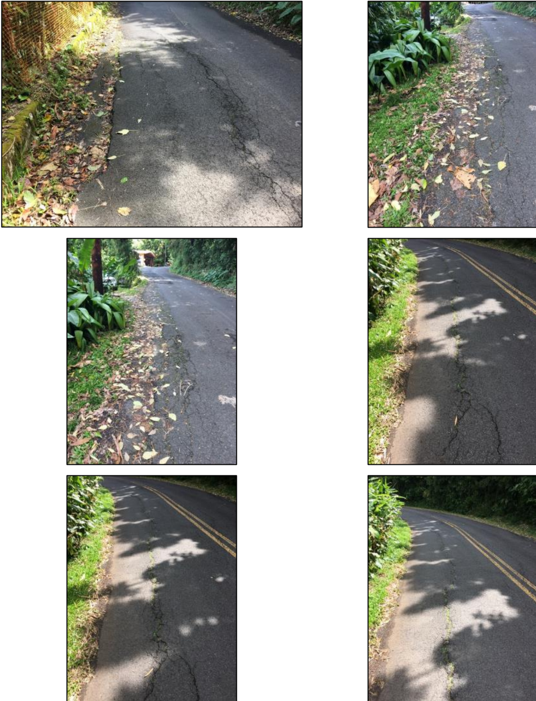
Figure 3.8 Subsidence Between 4110 Round Top Drive and Forest Ridge Way
