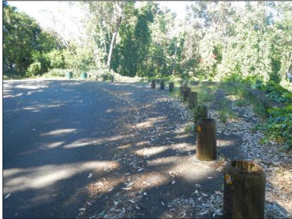
View of parking area T9.
