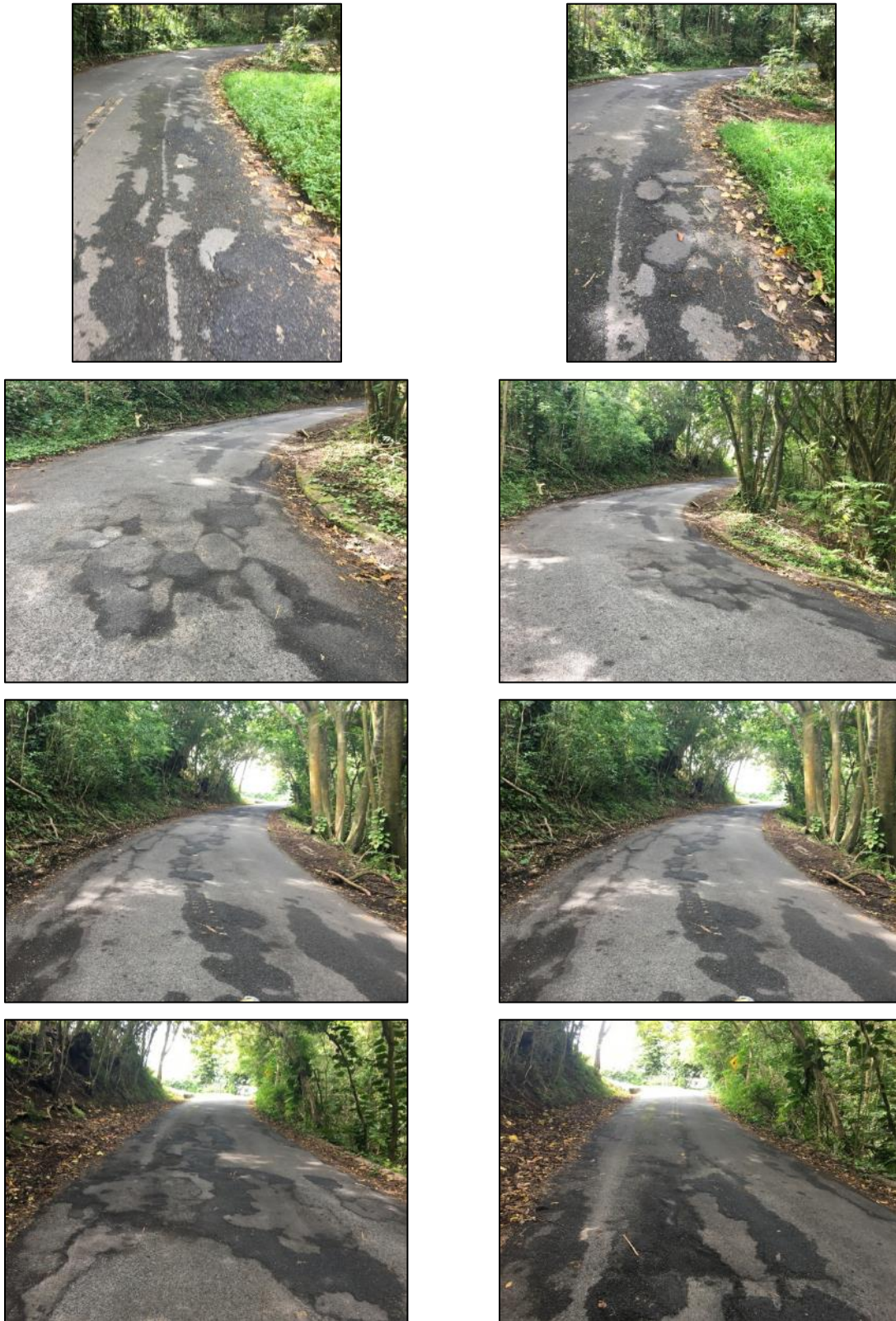
Figure 3.4 Existing Conditions in the Vicinity of 3200 Block of Round Top Drive
